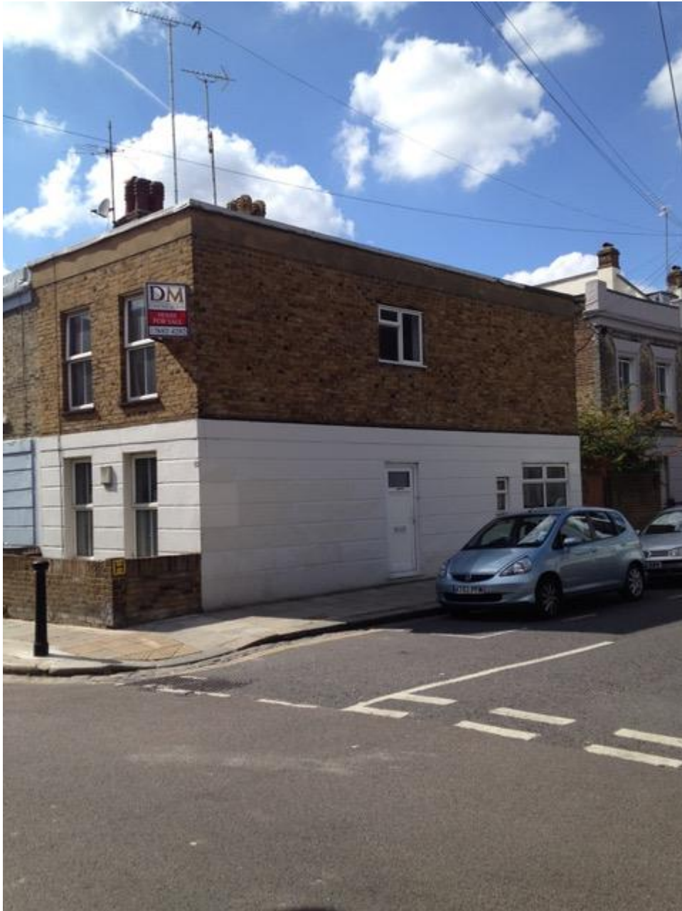
Figure 3 Side elevation facing Raglan Street
