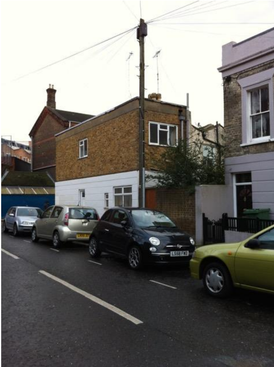
Figure 4 Side/rear elevation facing Raglan Street
