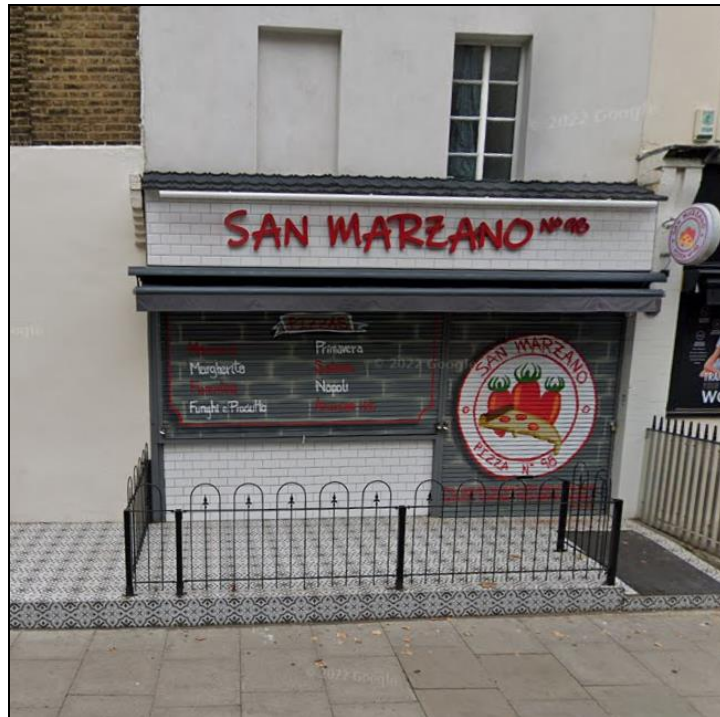
Figure 1: Former non-descript shopfront with solid metal shutters.
