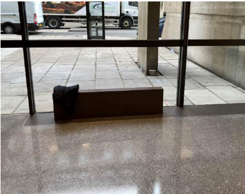
Rubber floor finish to radiator trench at L3 Atrium
