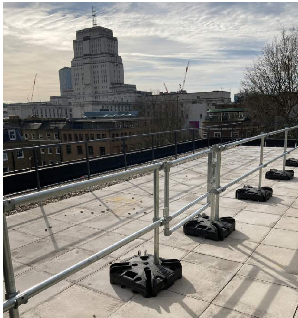
L9 Wing Terrace - new paving & temporary edge protection
