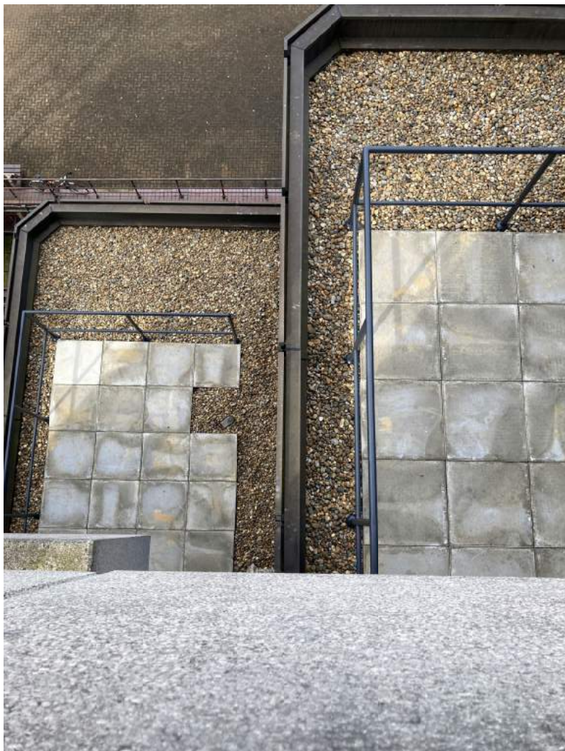
L6-8 – enhanced thermal roof finish
