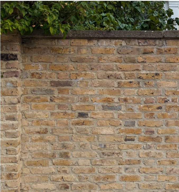
Reinstated wall at No.1 Fitzroy Rd.
