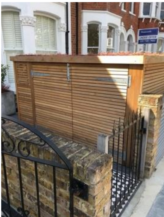
Photos of bin and bike store installed without permission
