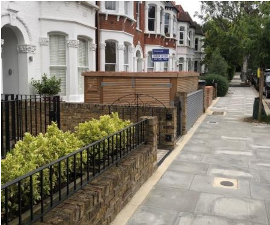
Photos of bin and bike store installed without permission
