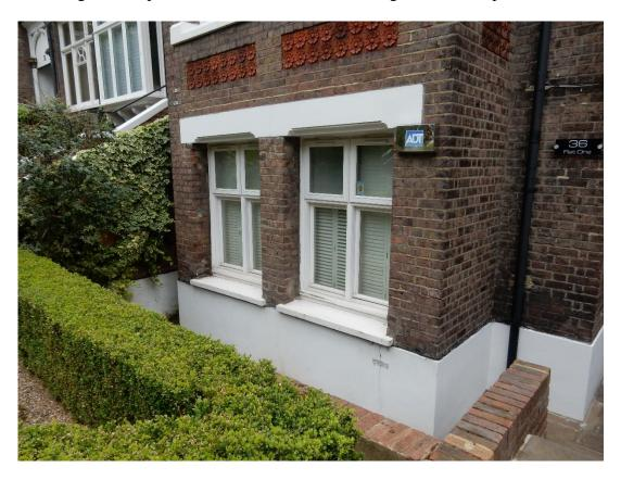
The painted timber windows to the right hand of the front elevation of Flat 1 have been distorted out of shape and alignment as a result of movement of the façade due to subsidence. The casements can no longer be opened as a result of this.
