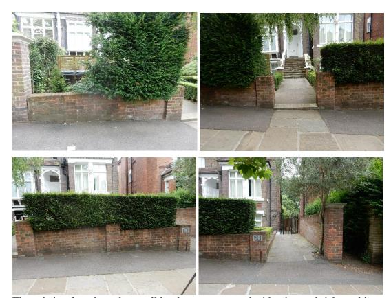
The existing front boundary wall has been constructed with wire cut bricks and is not original. It is also now weathered and out of the alignment.
