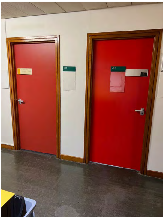
4 th Floor – pre refurbishment Office/teaching room decorated flush panel doors with stained hardwood frames, architraves & skirtings
