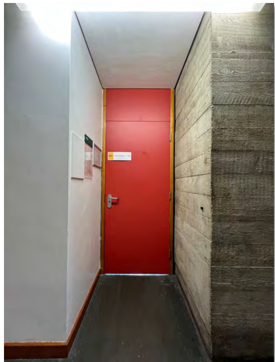
4 th Floor - pre refurbishment Office/teaching room later addition laminate faced flush panel door with fixed panel over
