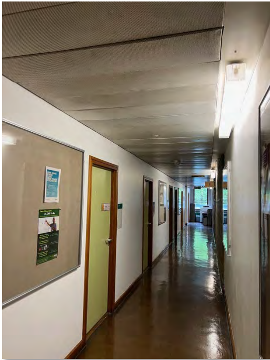
2 nd Floor Typical corridor view pre refurbishment Office/teaching room decorated flush panel doors with stained hardwood frames, architraves & skirtings
