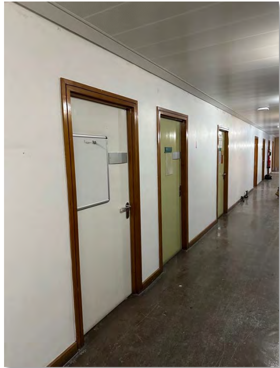
3 rd Floor Typical corridor view pre refurbishment Office/teaching room decorated flush panel doors with stained hardwood frames, architraves & skirtings
