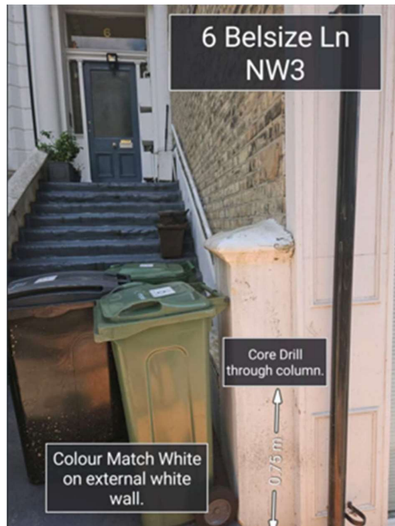
Figure 1 – Initial section of Gas Riser Pipework to be installed within the column located outside of the property, with connections to the handrail (painted white).
