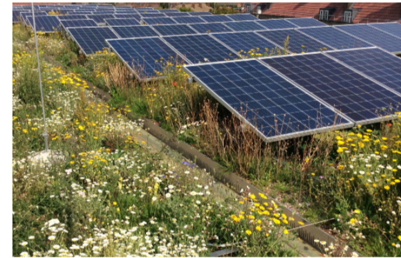
Extensive green roof
