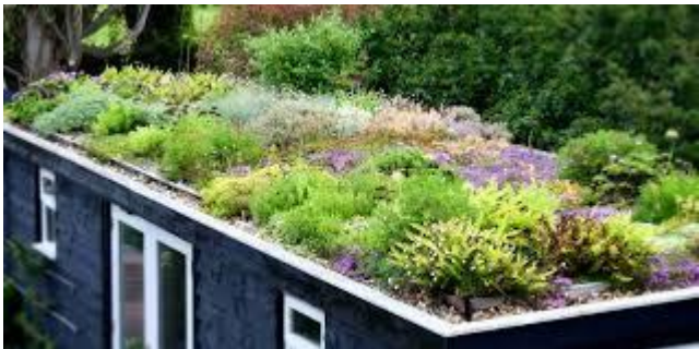
Figure 11: Example Green Roof
