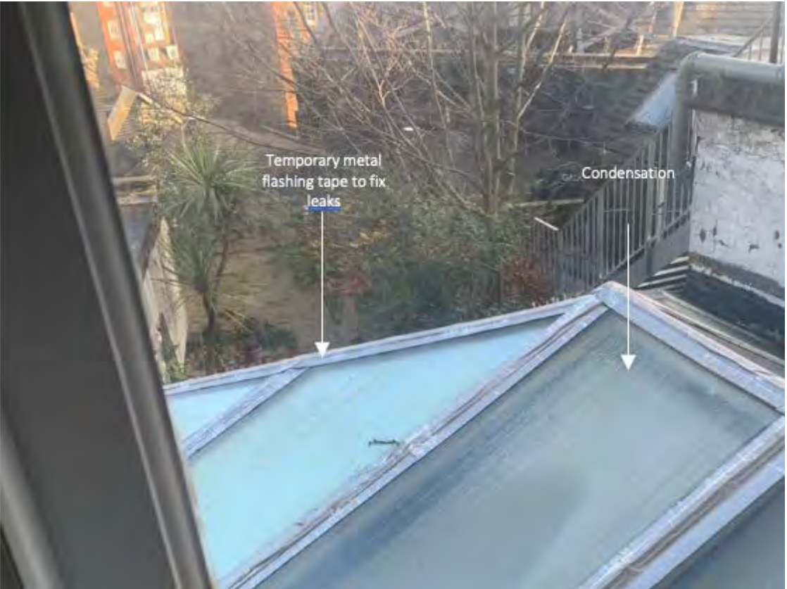
Figure 10. The existing rear conservatory is poorly insulated and ventilated and difficult to keep weatherproof (see temporary flashing tape) giving rise to condensation, mould and damp.
