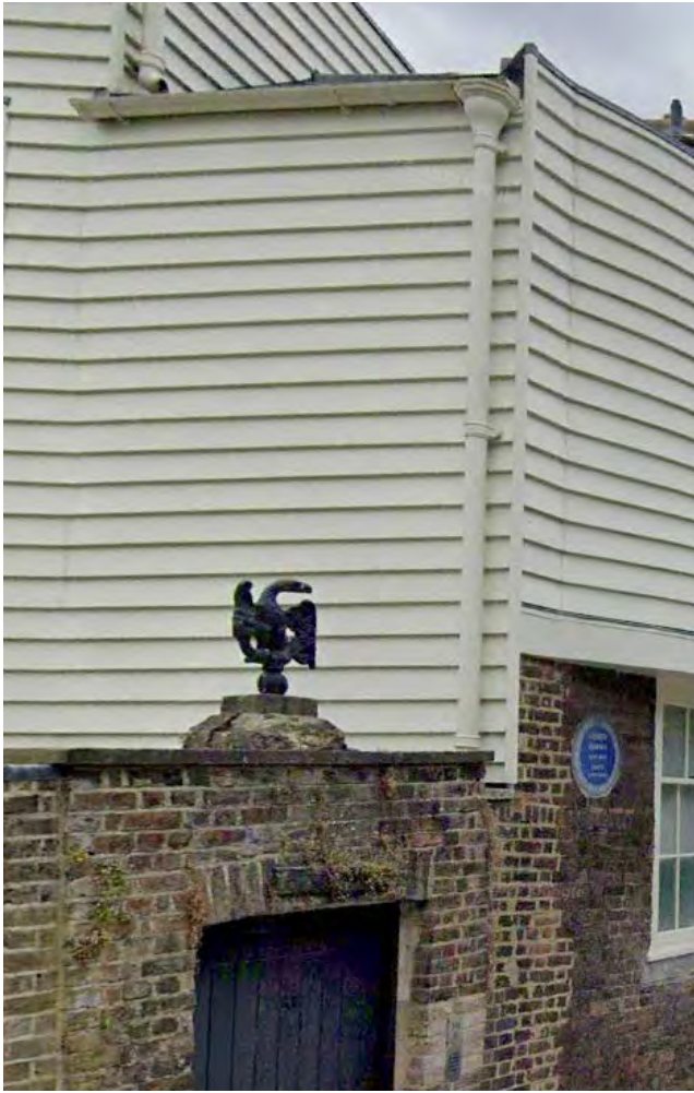
Figure 20. Traditional natural timber feathered cladding/ weatherboarding (Image: Google Earth)
