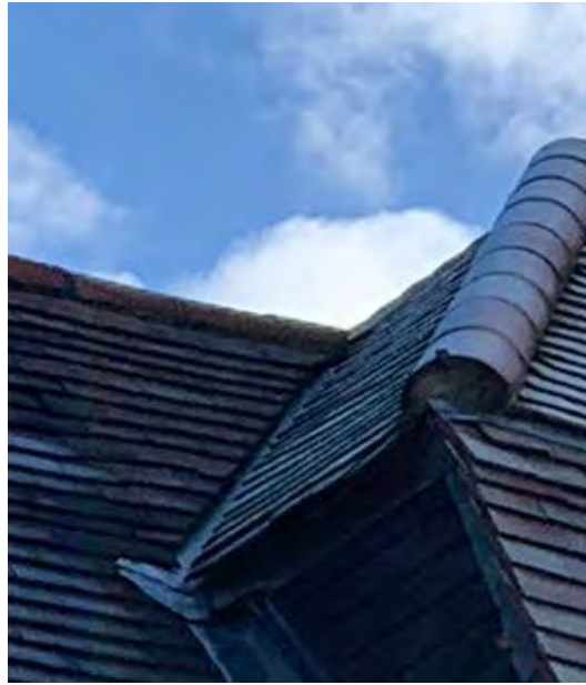
Figure 23. Existing plain tile roof with half-round clay ridge tiles and timber weatherboarding to the front flank elevation.
