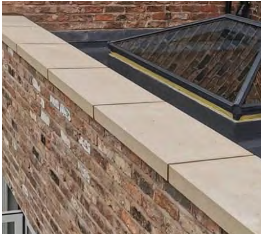
Figure 21. Parapet detail with stone coping
