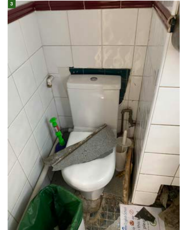
Figure 18. Existing WC within 47 BS.
