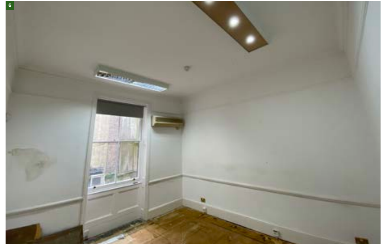
Figure 14. Existing back room within 47 BS.
