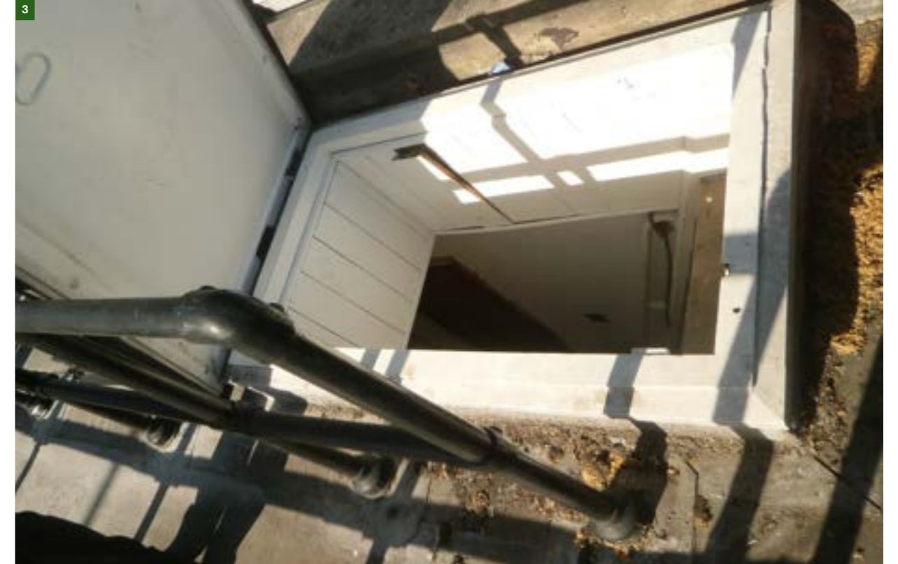
Figure 34. Access from 4th floor.
