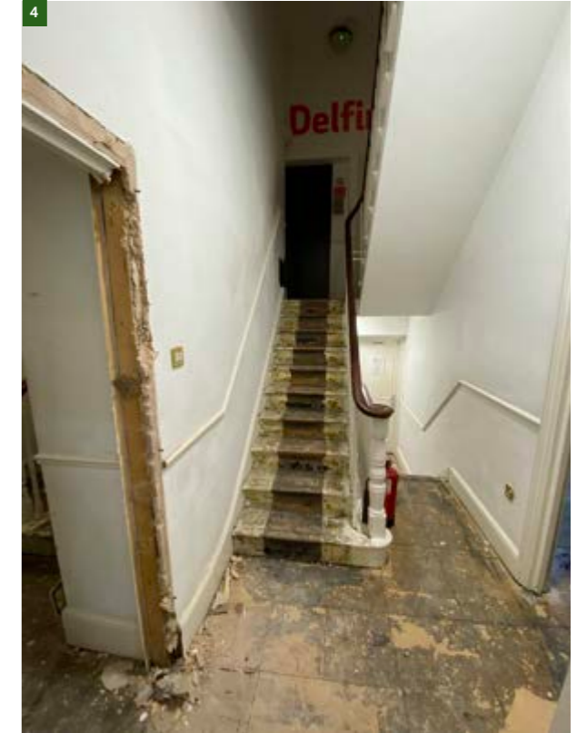
Figure 15. Existing stairs within 47 BS.
