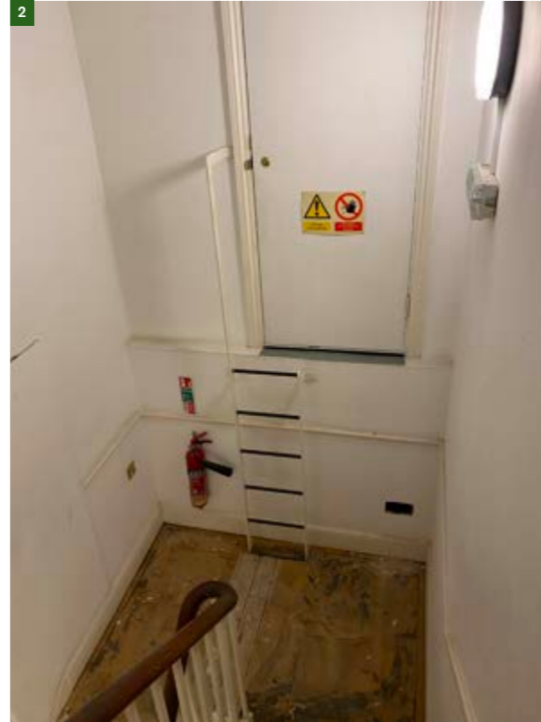
Figure 28. Access to lift plant room.
