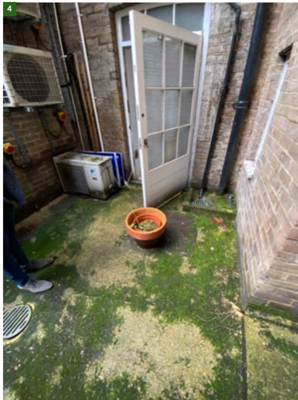
Figure 19. Lower ground courtyard within 47 BS.
