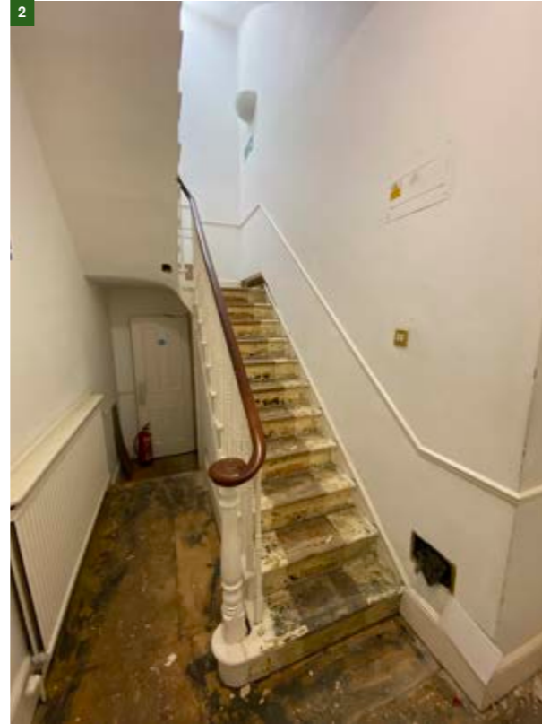
Figure 11. Existing stairs within 46 BS.
