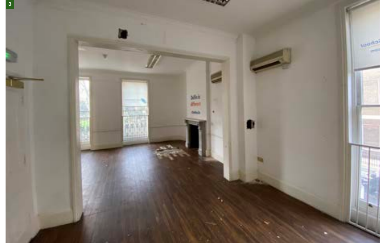
Figure 24. First floor front room within 47 BS.
