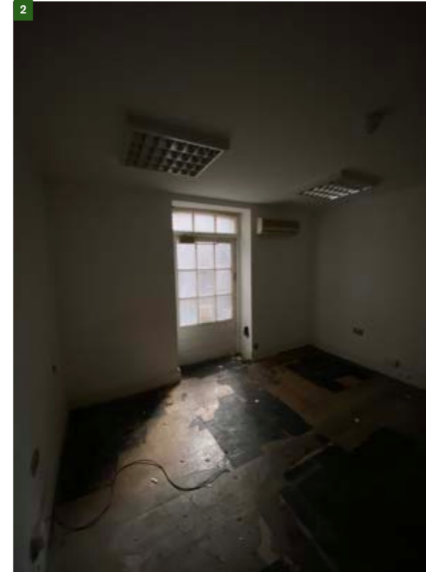
Figure 17. Rear room within 47 BS.
