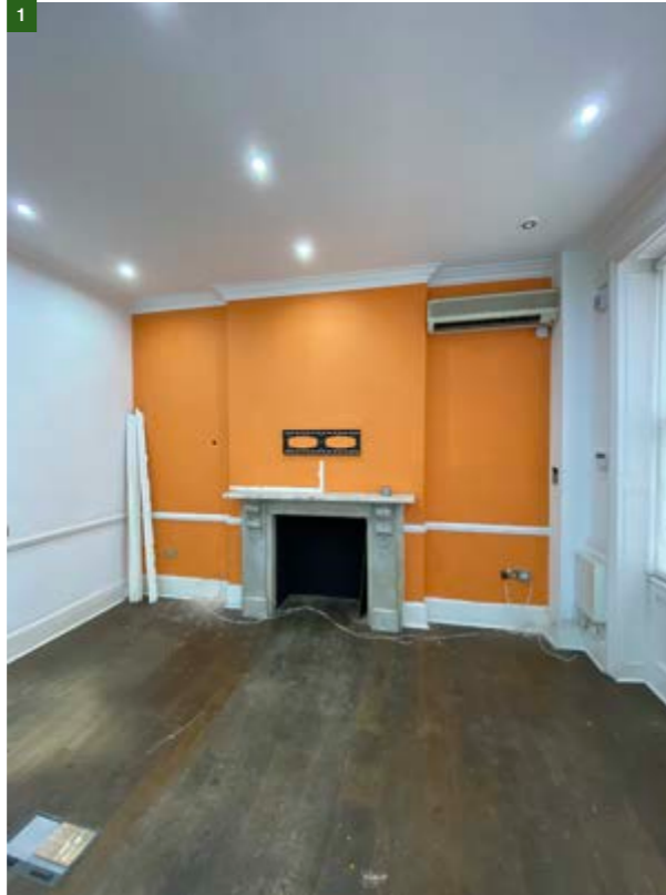
Figure 10. Existing front room within 47 BS.
