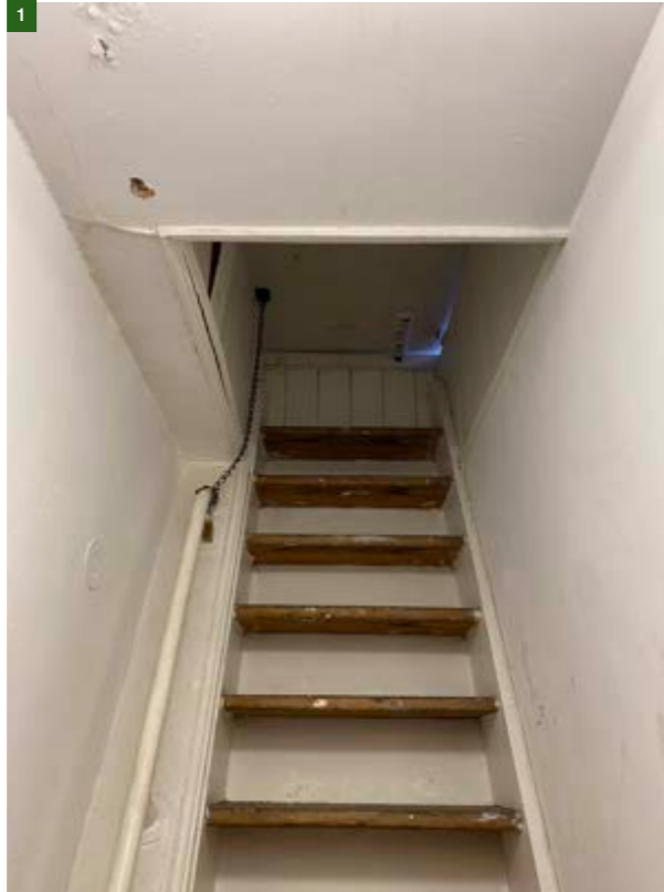
Figure 27. Access to roof.
