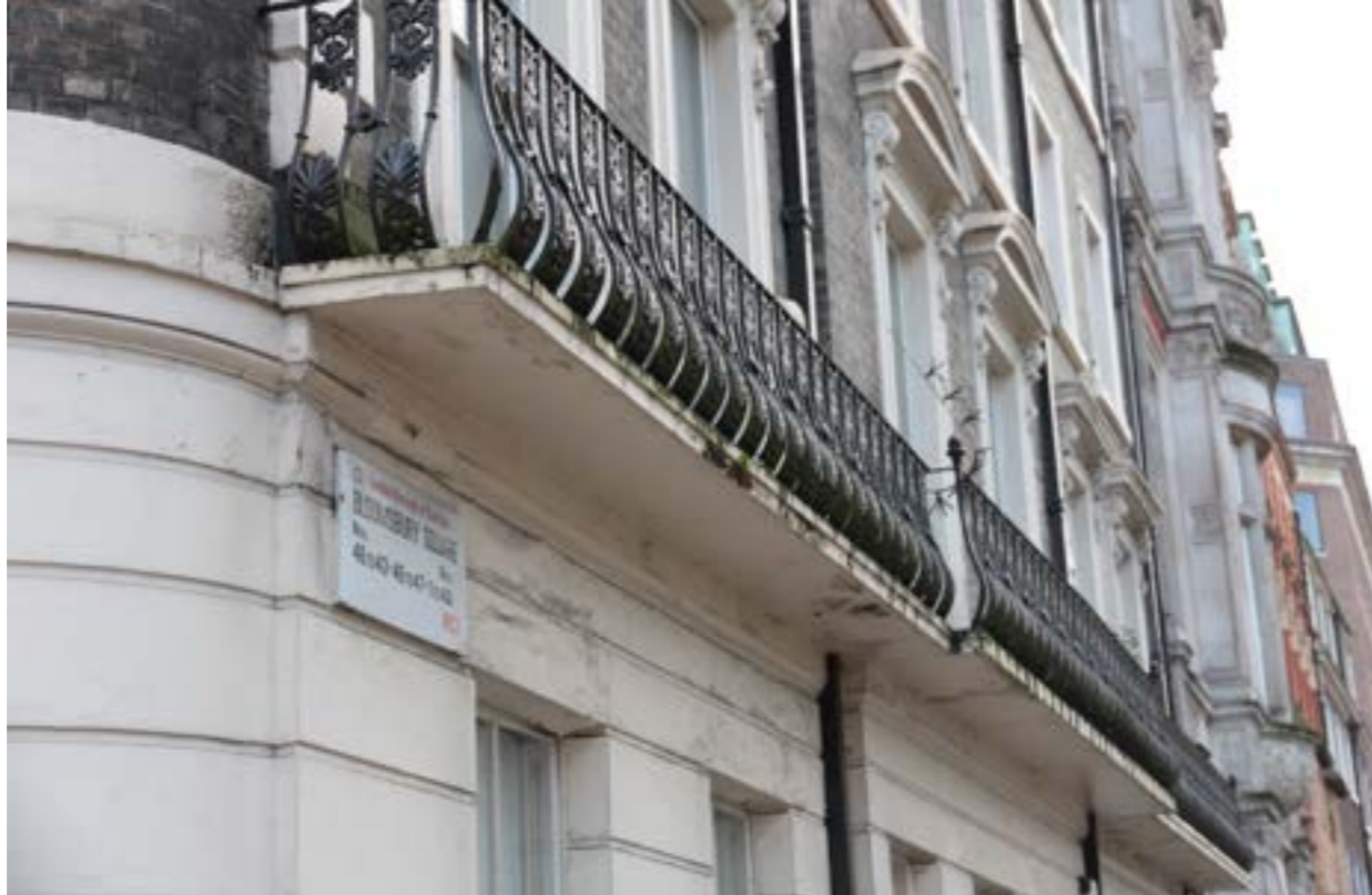
Figure 5. Existing balconies along Bloomsbury Square frontage.
