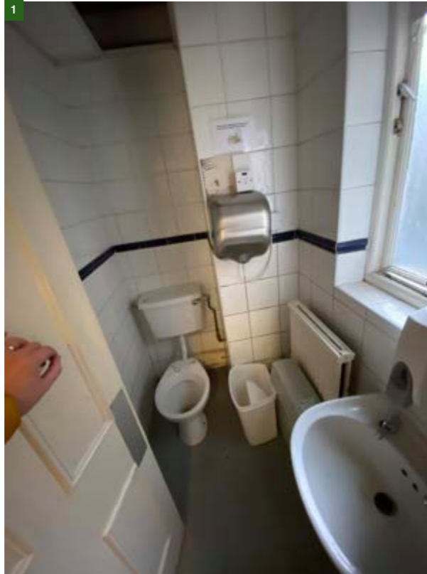
Figure 22. Example of existing WCs.
