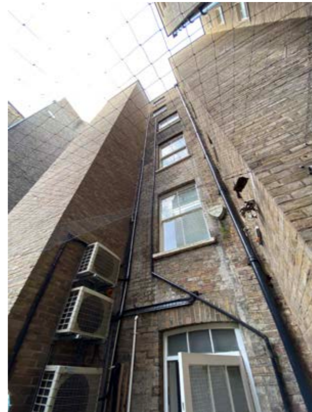
Figure 3. Rear of 47 BS showing modern extensions and plant.
