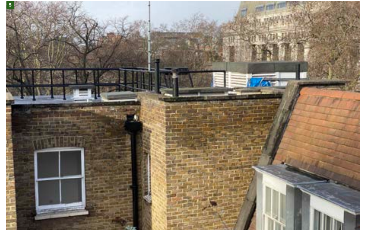
Figure 36. View onto roof from 22 Southampton Place.
