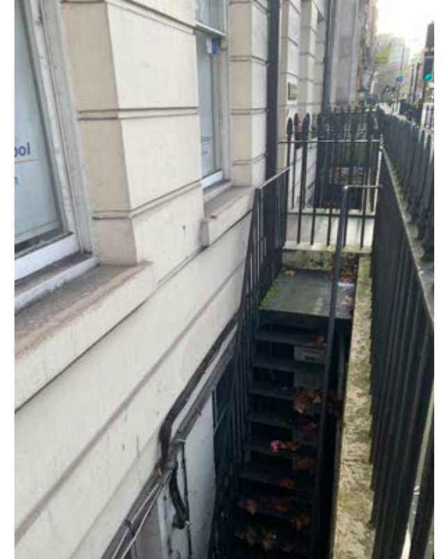
Figure 7. Stair access to lower ground.
