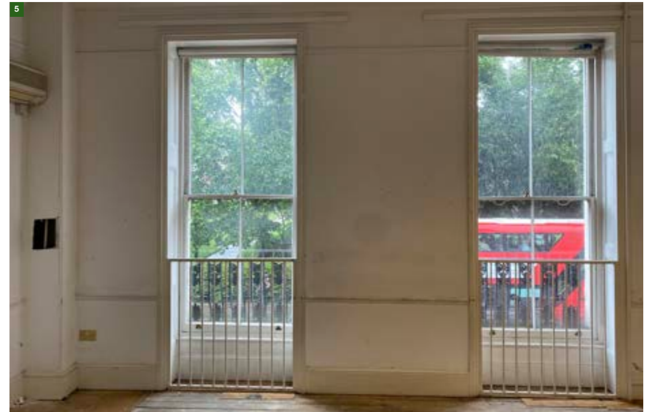
Figure 26. First floor windows and gaurding.
