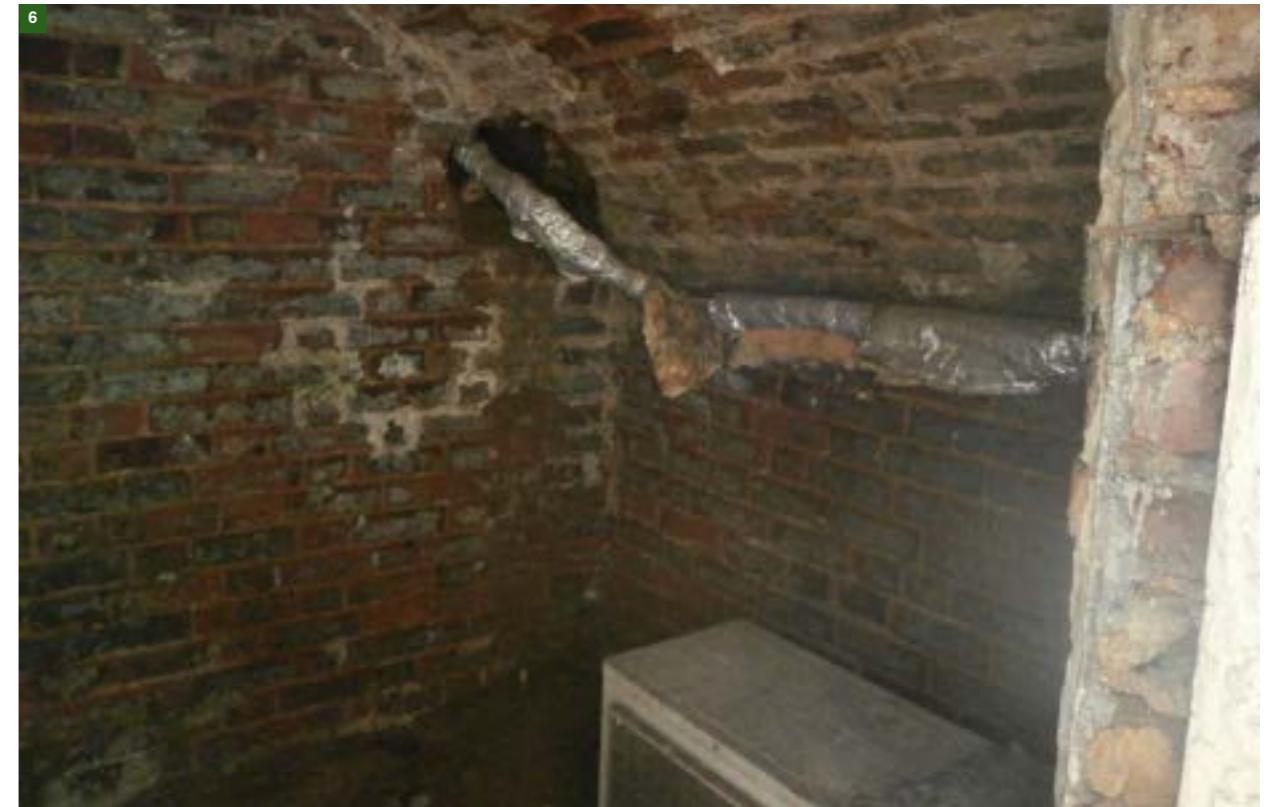
Figure 21. Lower ground vaults in front of 47 BS under Bloomsbury Square.
