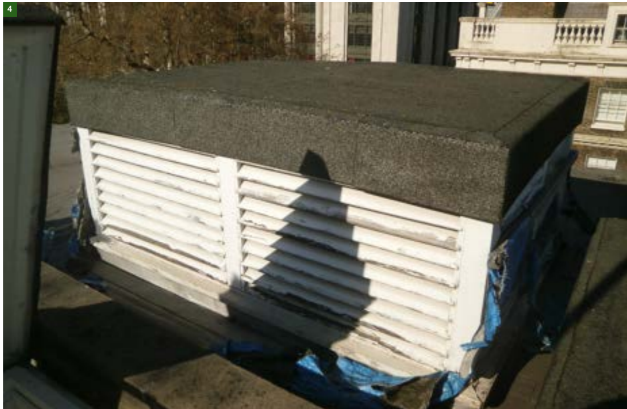
Figure 35. Existing cowl over plant room.
