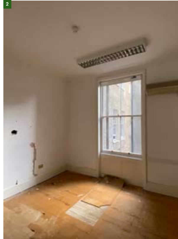
Figure 23. First floor back room within 47 BS.
