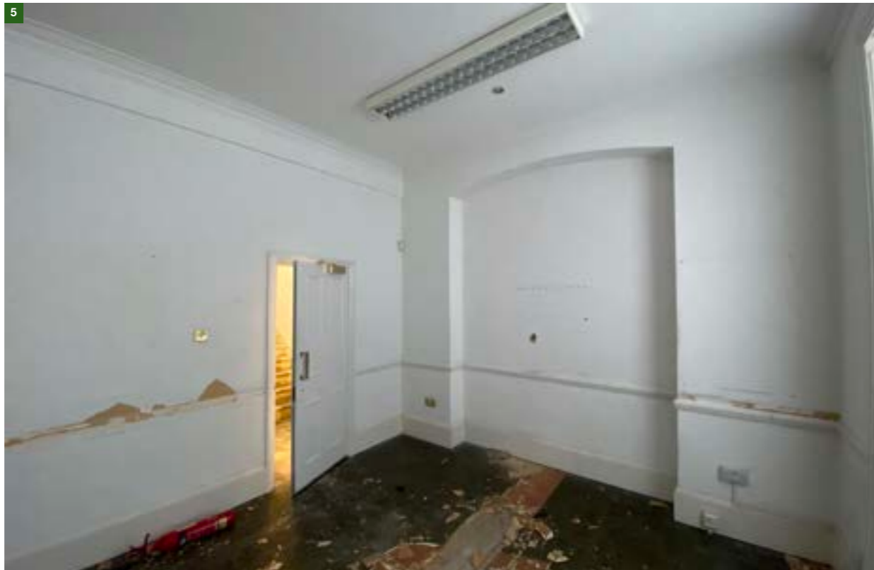
Figure 13. Existing front room within 47 BS.
