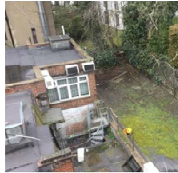
Garden to the rear of the existing building
