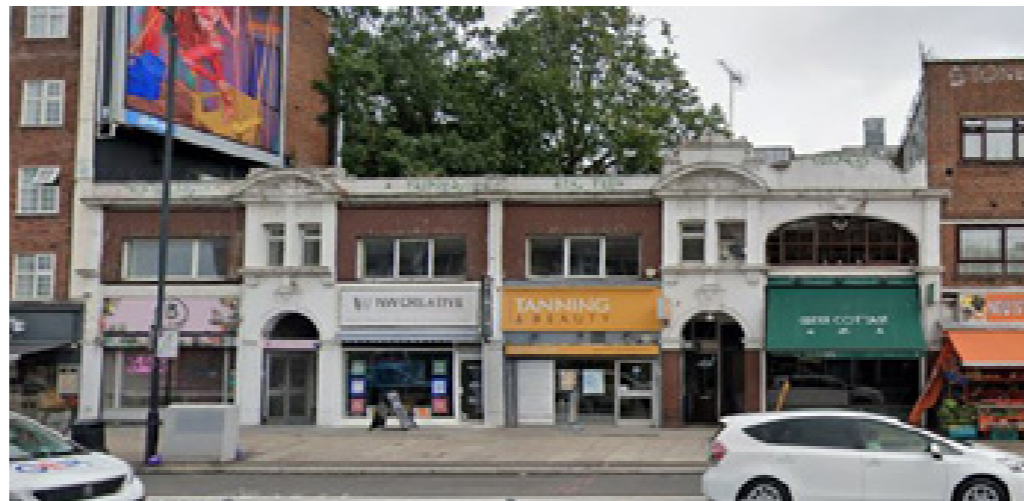
Existing front facade
