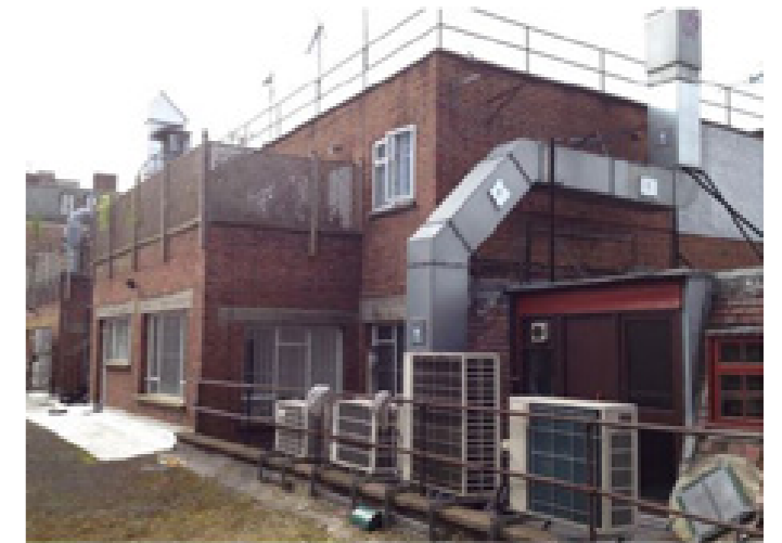
Rear of the existing building with neighbour in background
