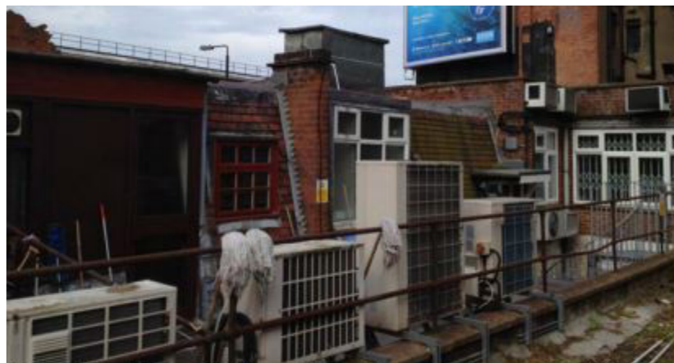
Rear of the existing building at second floor level
