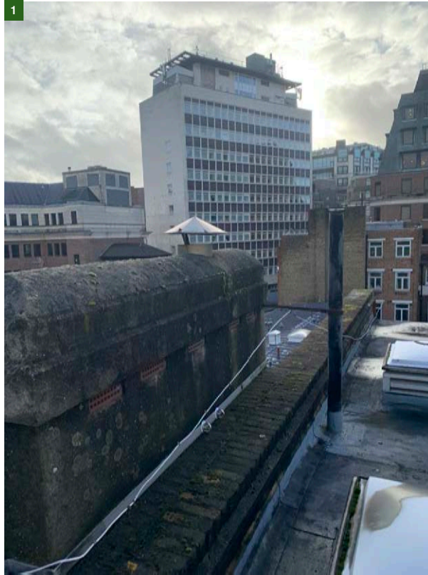
Figure 12. Existing capped chimneys.
