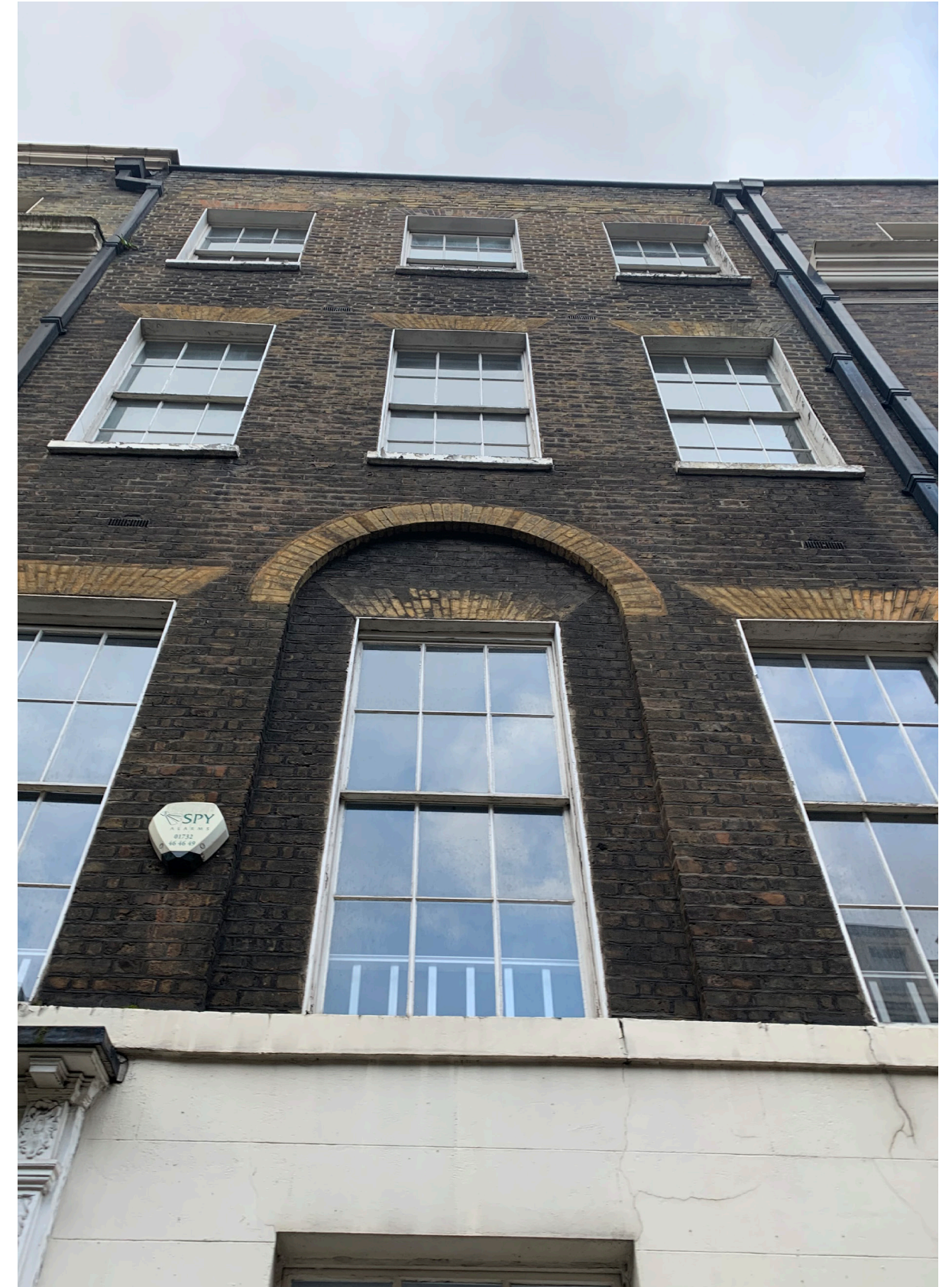
Figure 5. Main facade of 22 Southampton Place.
