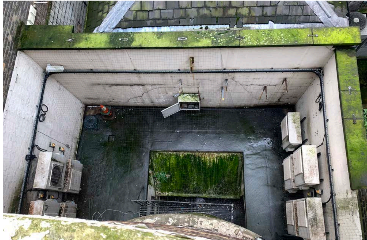
Figure 4. Rear of 22 Southampton Place.
