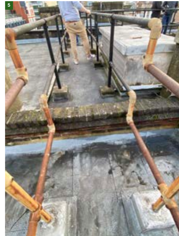
Figure 18. Access between 21 and 22 SP over party wall.
