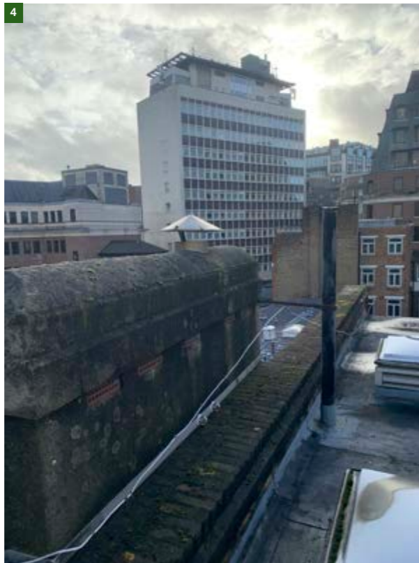
Figure 17. Existing capped chimneys.
