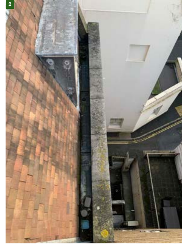
Figure 15. Existing gutters, mansard and dormers on 20 SP.
