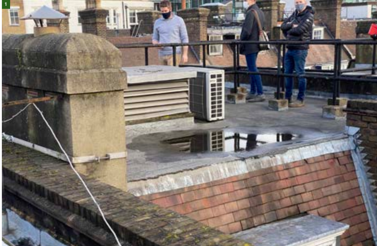
Figure 14. Existing roof on 21 SP.
