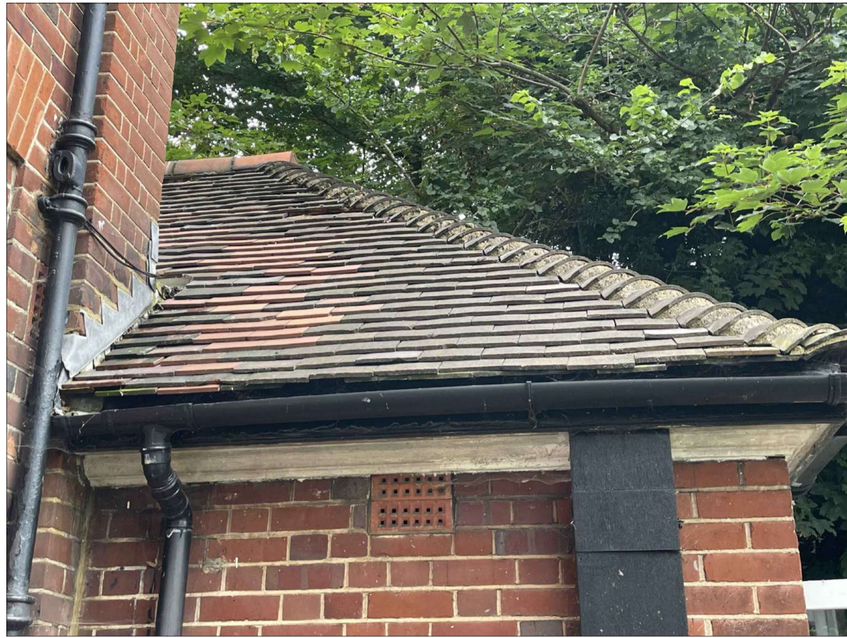
Image 2 - View of existing extension Roof from the rear garden
