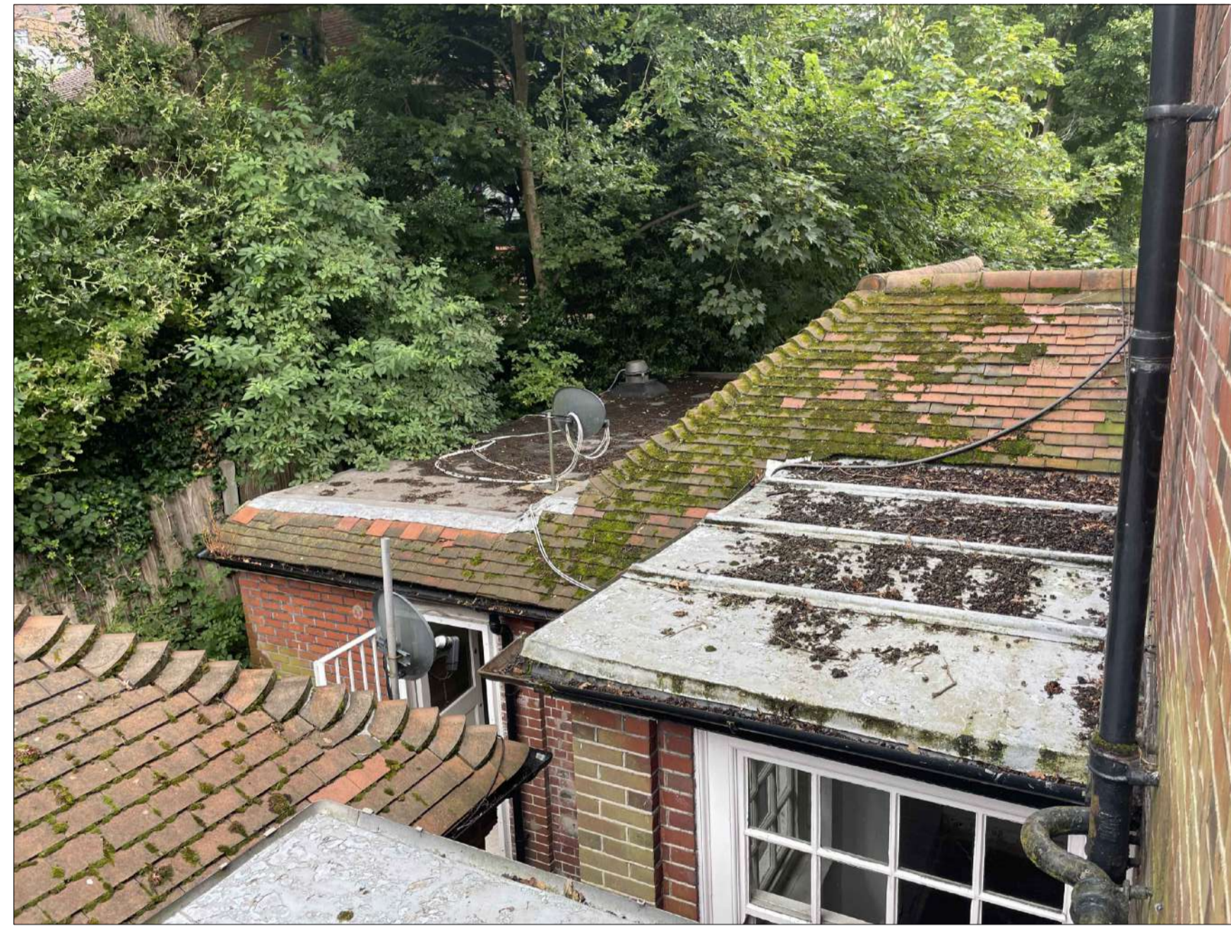
Image 3 - View of existing extension Roof from the side of the house
