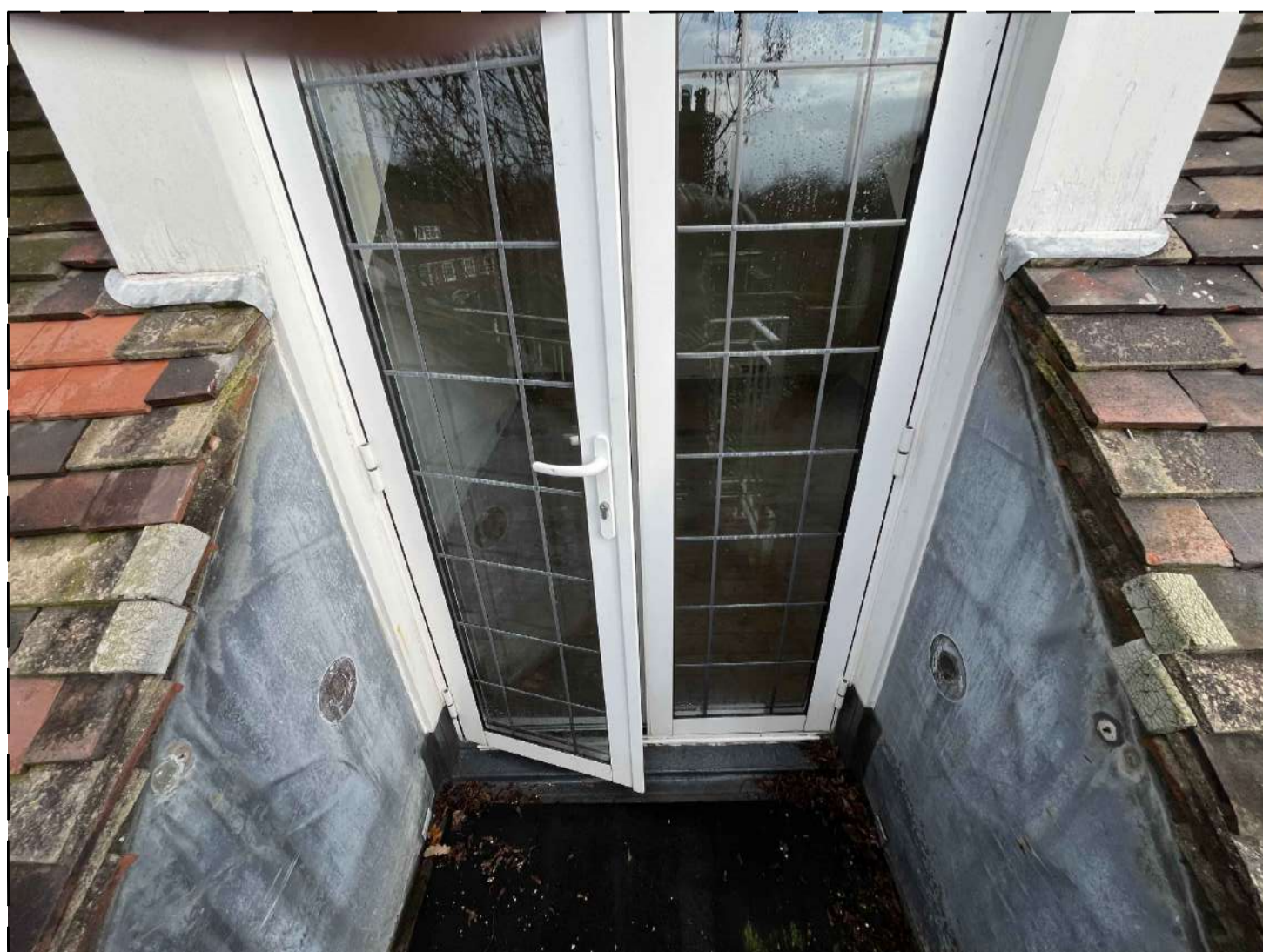
Image 5 - View door dormer Roof detail at 2nd floor
