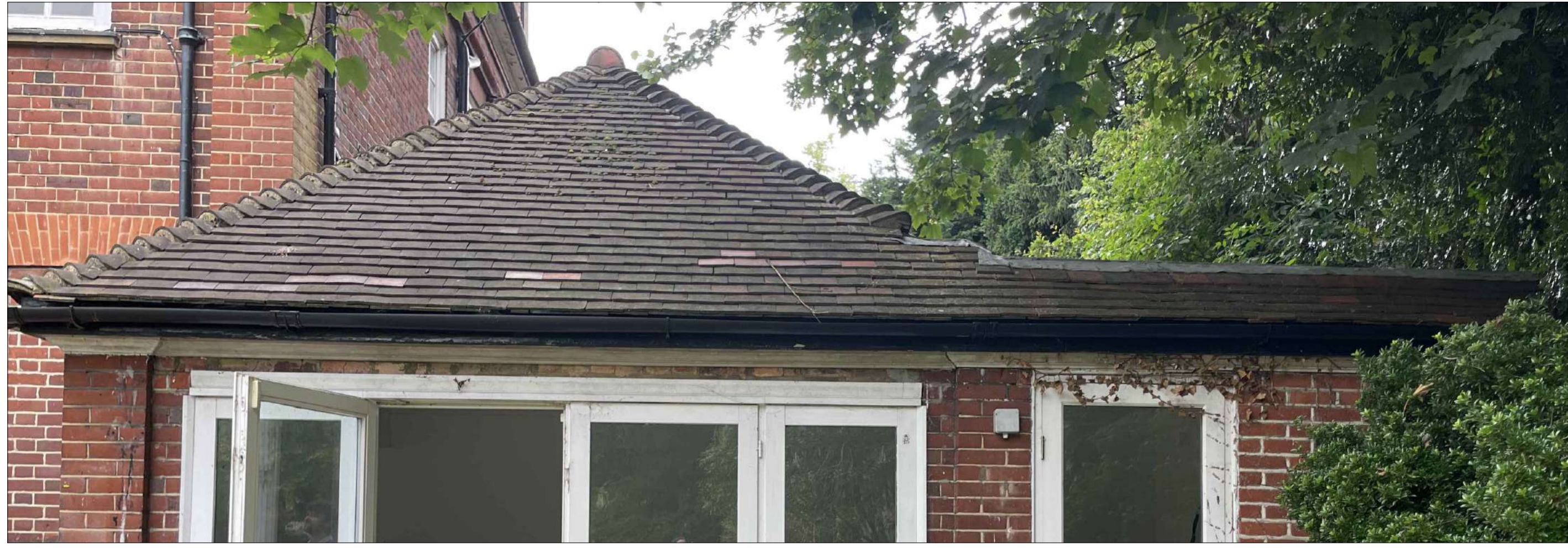
Image 1 - View of existing extension Roof from the rear garden
