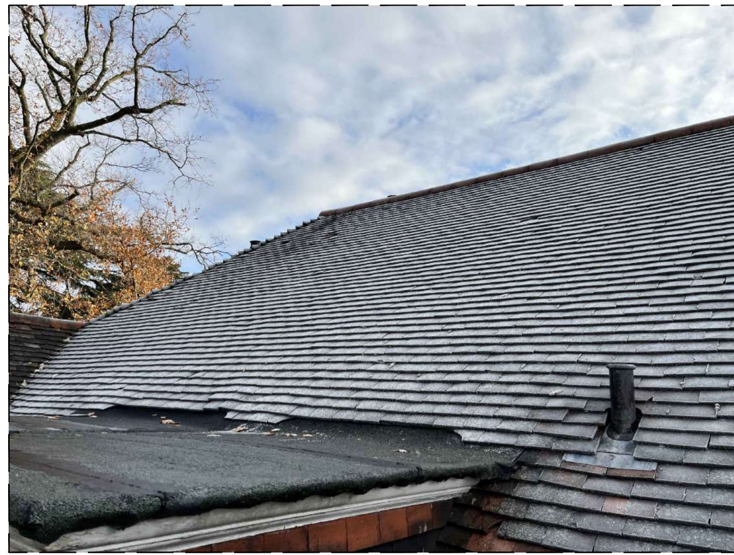
Image 2 - View of existing Roof from the terrace at 2nd floor
