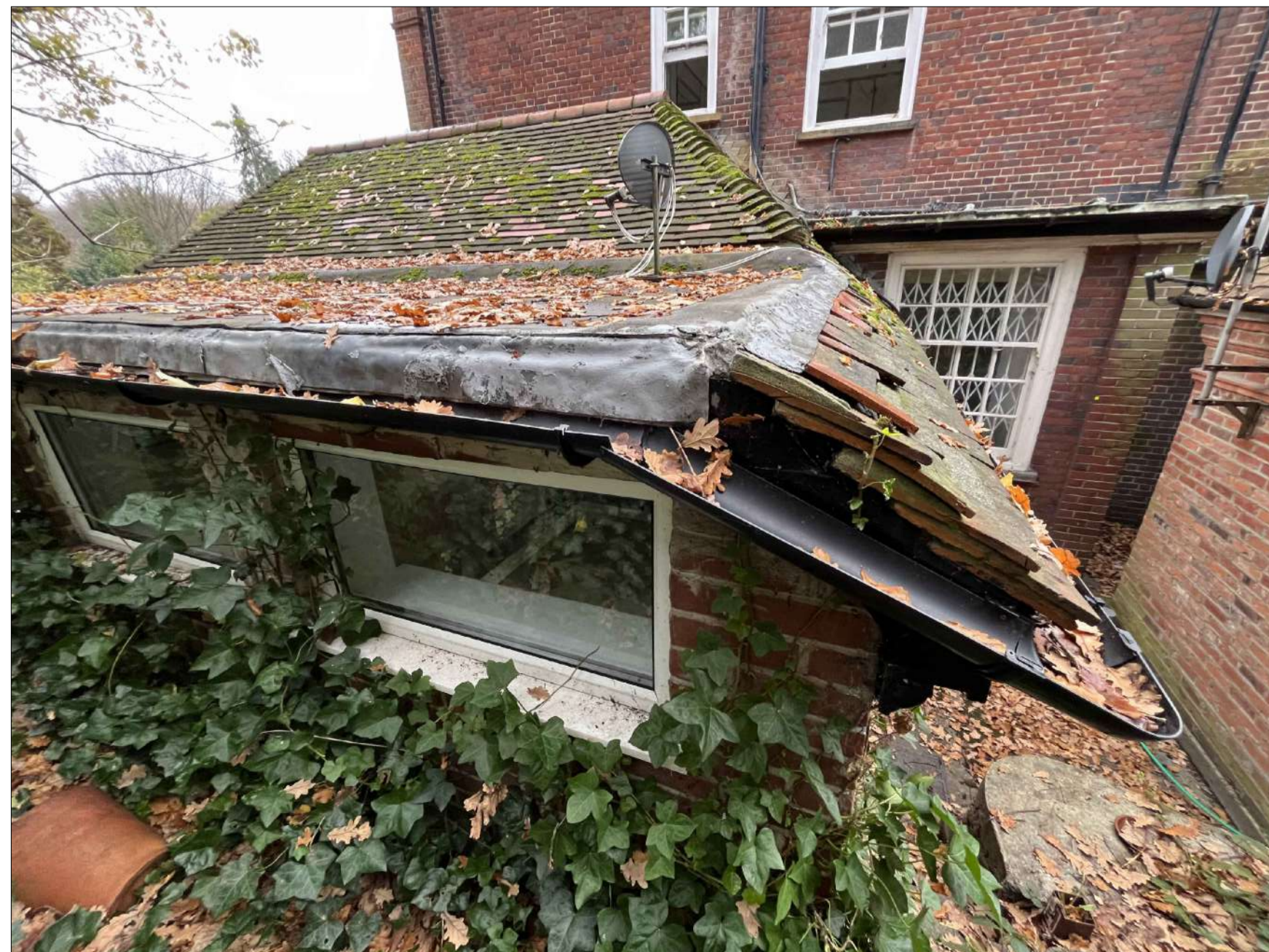
Image 5 - Side view of existing extension Roof
