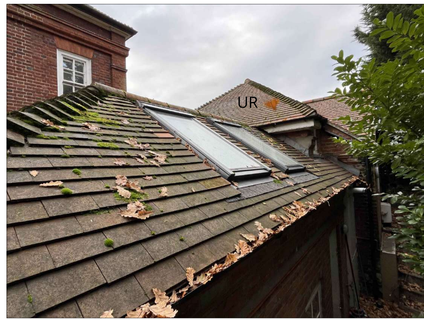
Image 2 - Side View of existing Coach House
