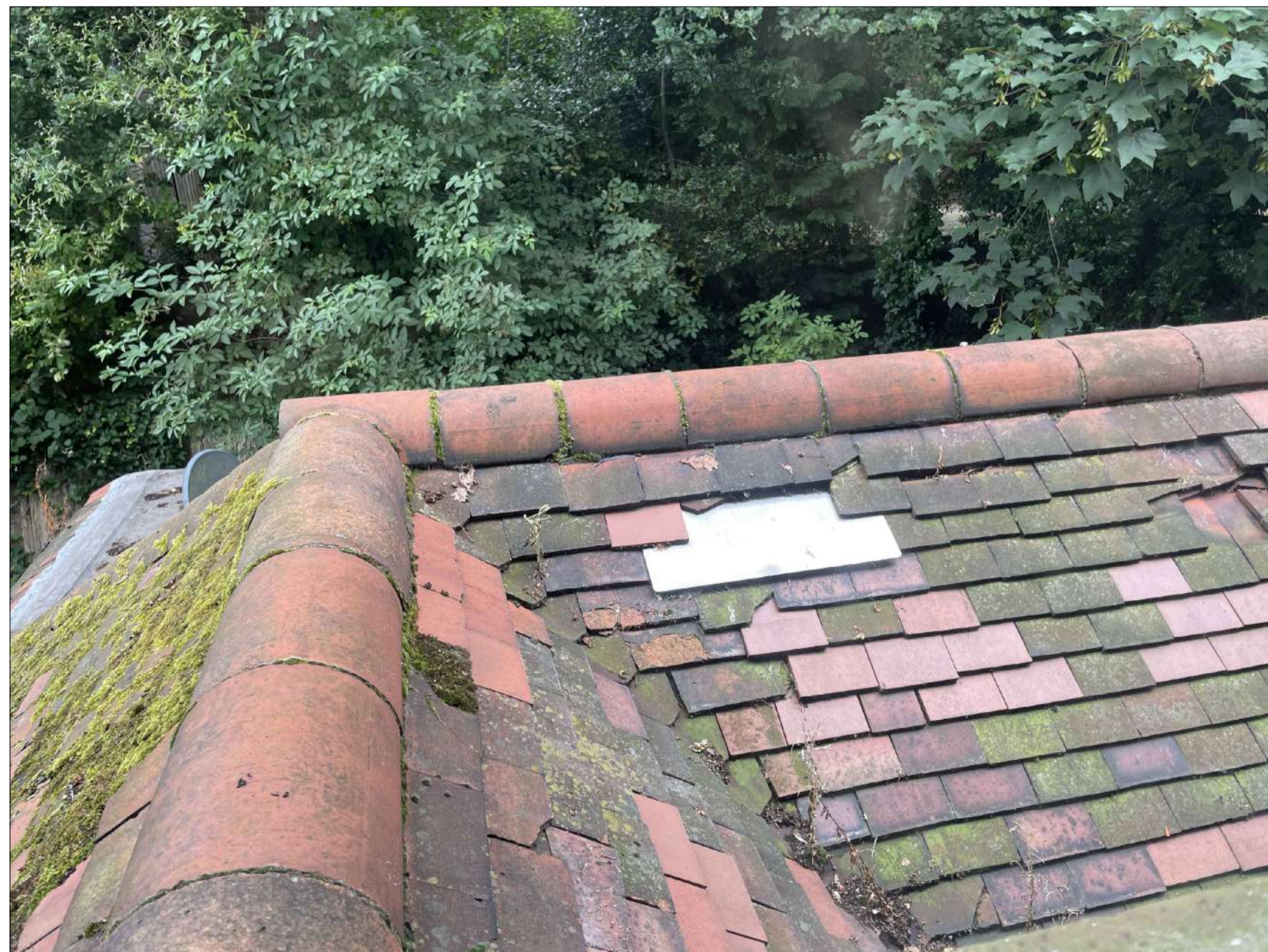
Image 4 - Roof View of existing Roof detail
