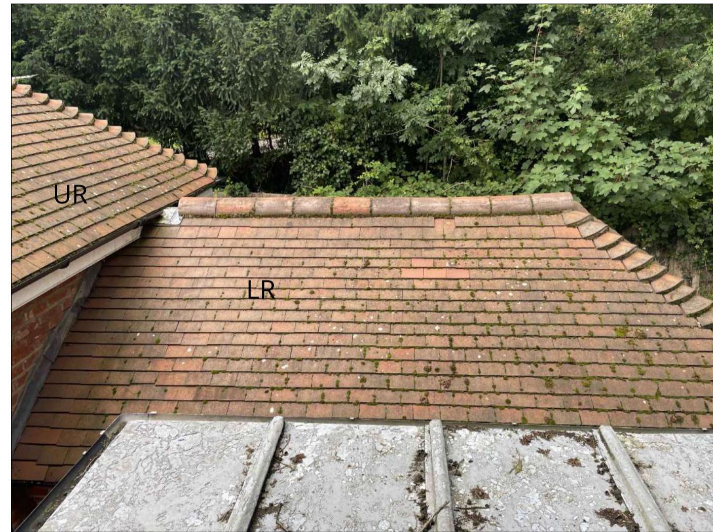
Image 4 - View of rear coach house roofs junctions
