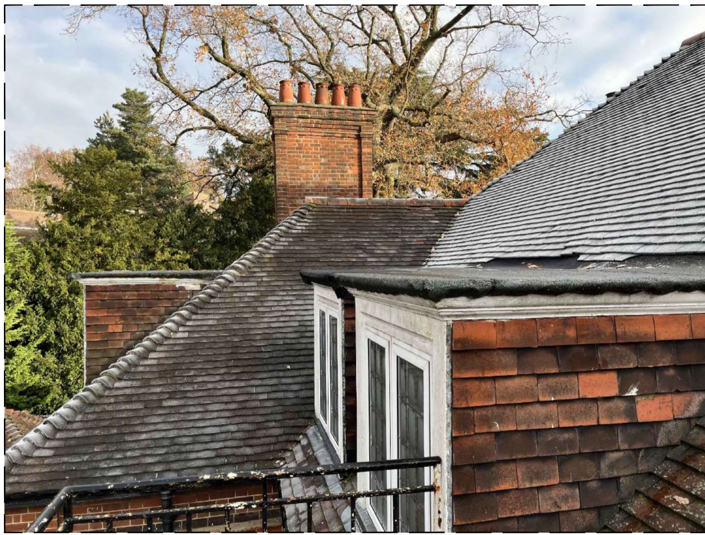
Image 1 - View of dormer windows and roof
