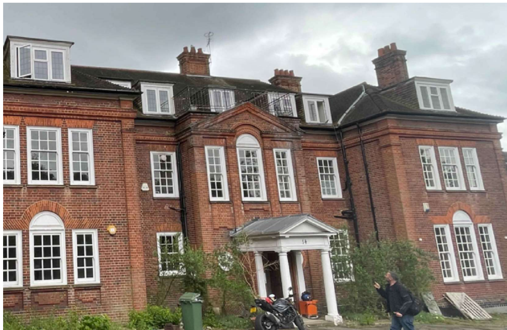
Image 3 - General front view of the main house roof
