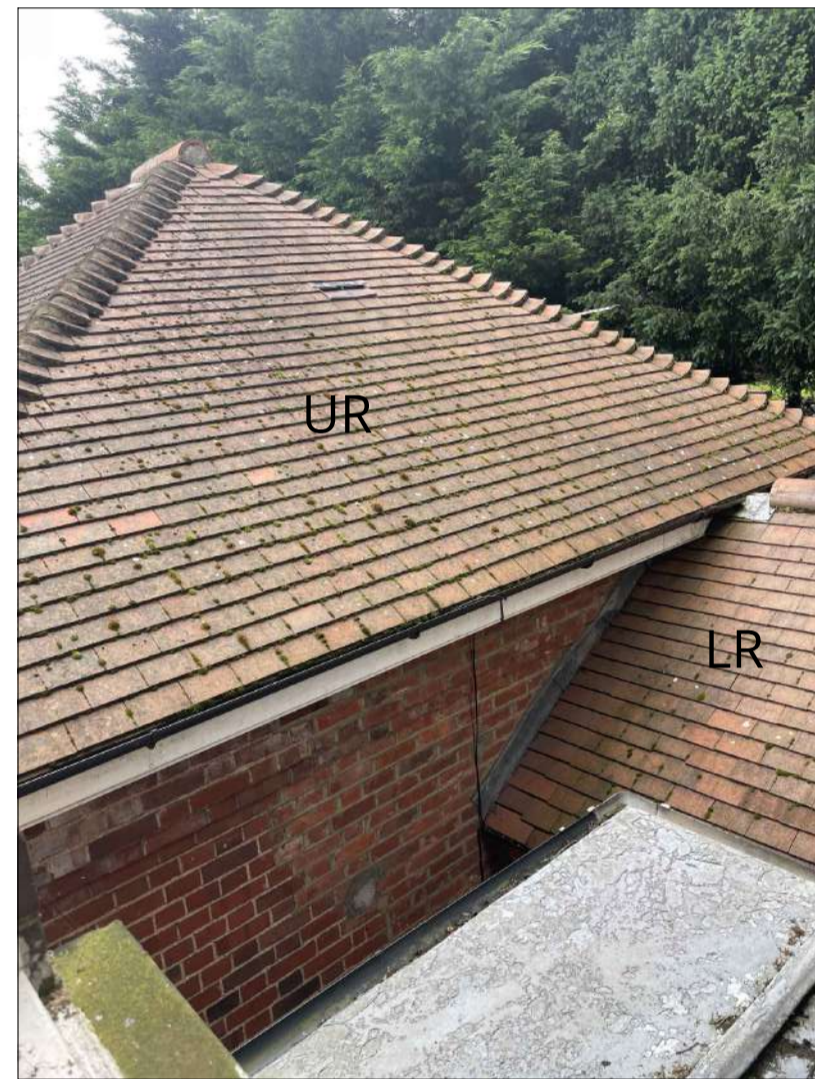
Image 3 - View of rear coach house roofs junctions
