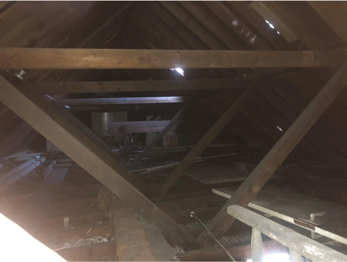
Figure 14: Timber roof structure.
