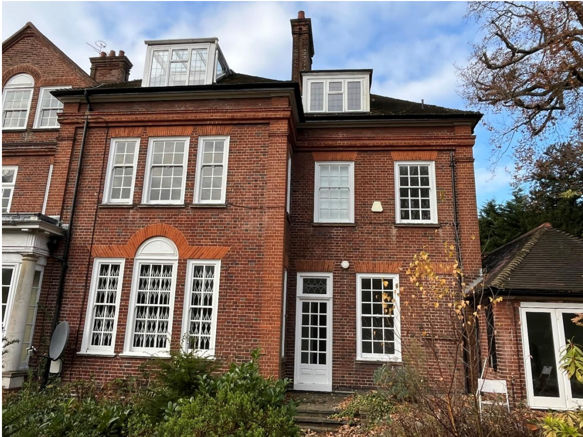
Figure 13: View of the fully glazed dormer at the rear.
