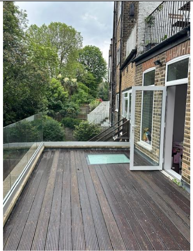
Fig.6. Photographs of the rear erected terrace and glass balustrade
