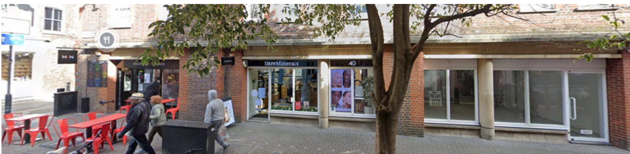
Photo 2 (above): Street View, Neal Street Elevation (source: Google 3D)
