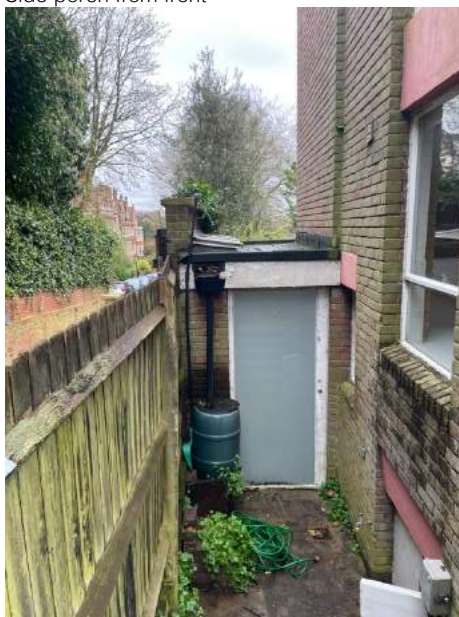
q. Side porch from rear
