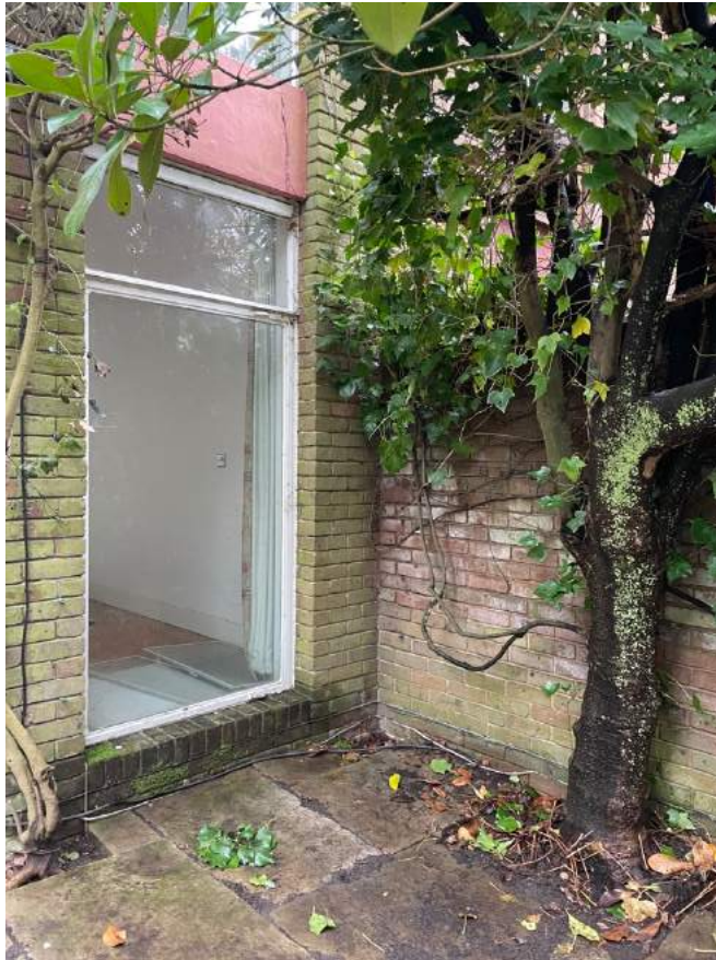
l. Rear – boundary wall between 18A and 18B
