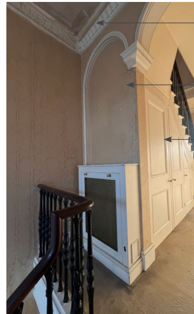
PHOTO OF TOP OF MAIN STAIR
