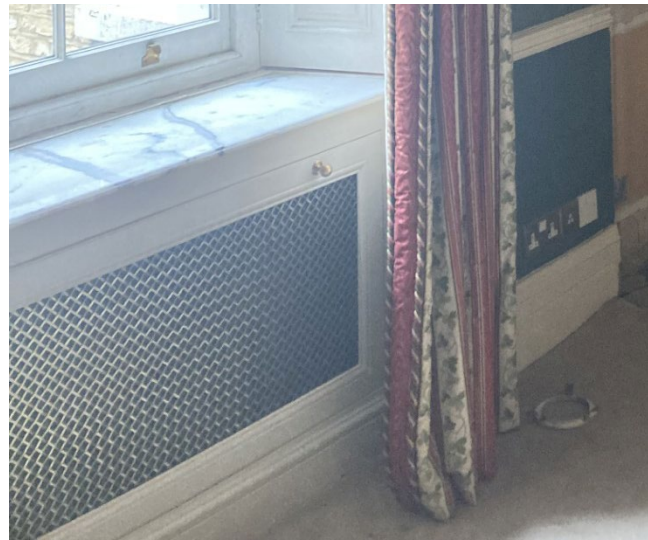
PHOTO OF EXISTING CONDITION
