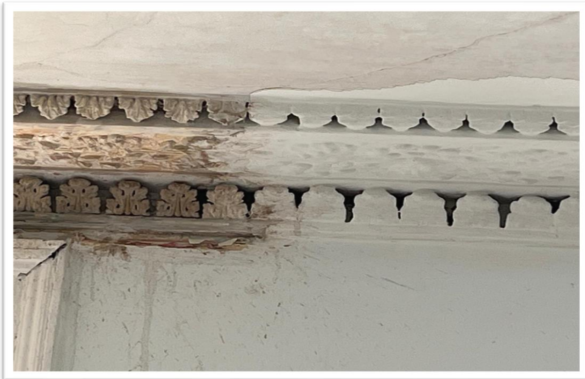
Photo 2-after paint stripping the decorative atheneum leaves de-bonded, which were carefully reconnected.
