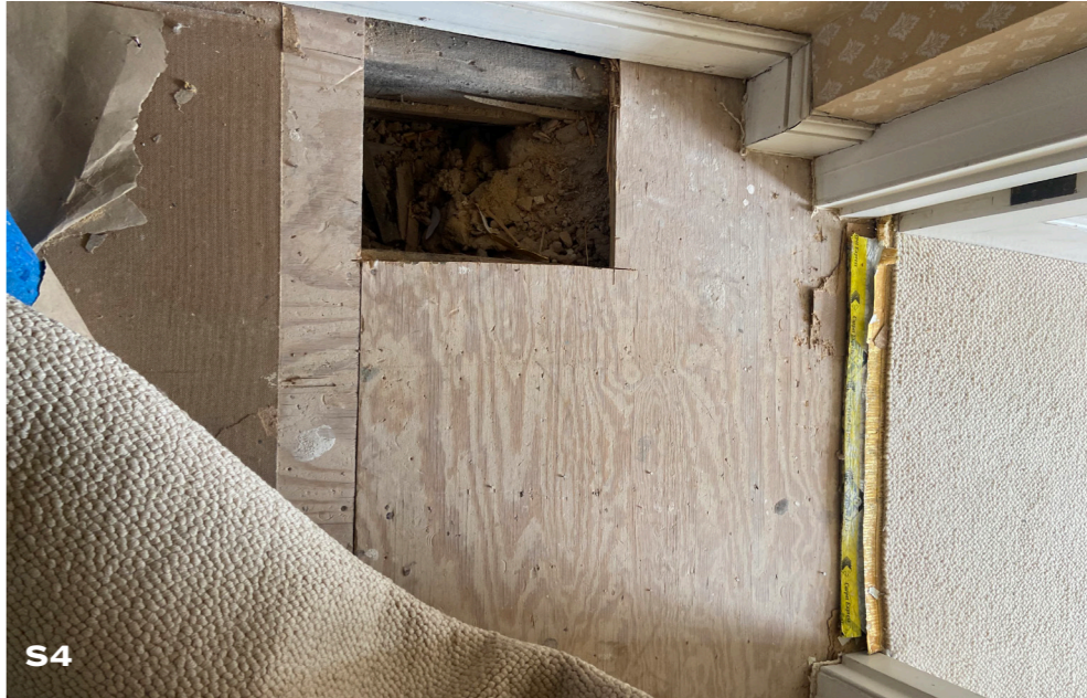
S4 Master Dressing Room (33) Carpeting and underlay were lifted up, showing plywood boarding on joists.
