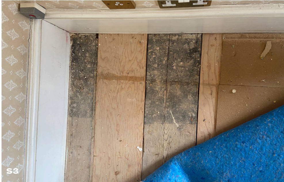
S3 Master Bedroom (34) Carpeting and underlay were lifted up, showing cut floorboards and modern inserts.
