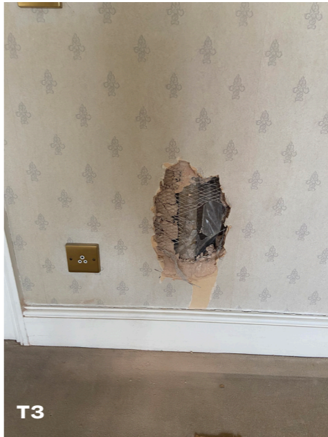
T2 Third Floor Bedroom (41/39) Opening reveals walls are made of timber battens with EML mesh and plaster.
