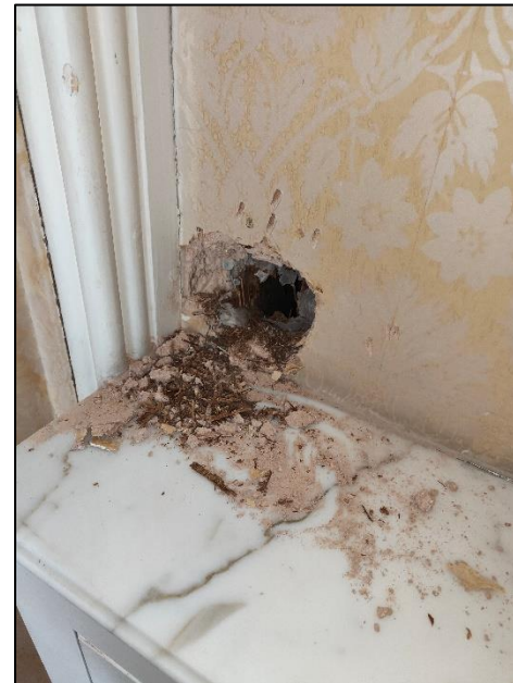
SECOND FLOOR SW1 Plaster on timber studwork partition
