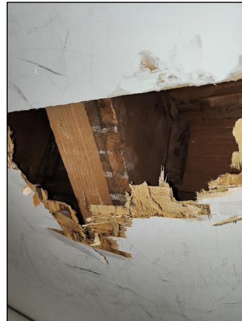
THIRD FLOOR STAIR Timber boarding on stair soffit
