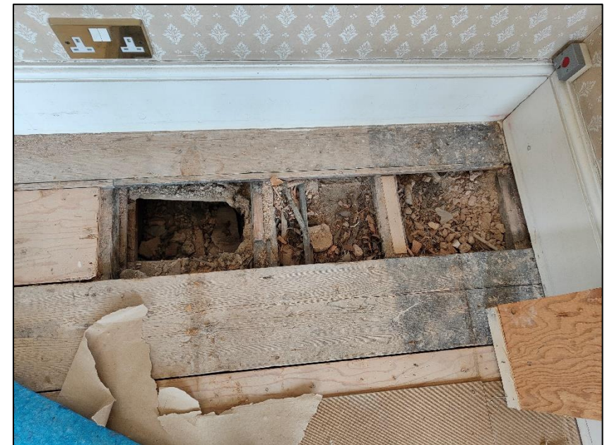
SECOND FLOOR S1 Timber boarding on timber joists with pugging
