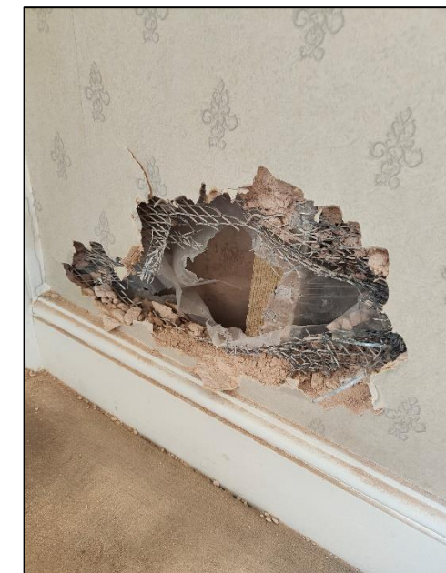
THIRD FLOOR TW1 Plaster on metal lathe on timber studwork
