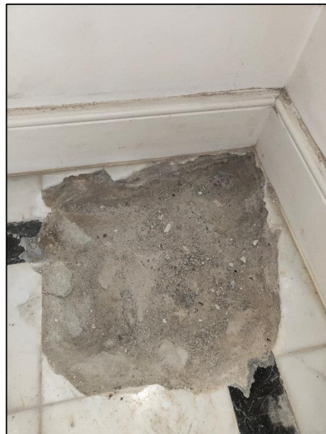
LOWER GROUND FLOOR TP5 Concrete slab (depth not determined)
