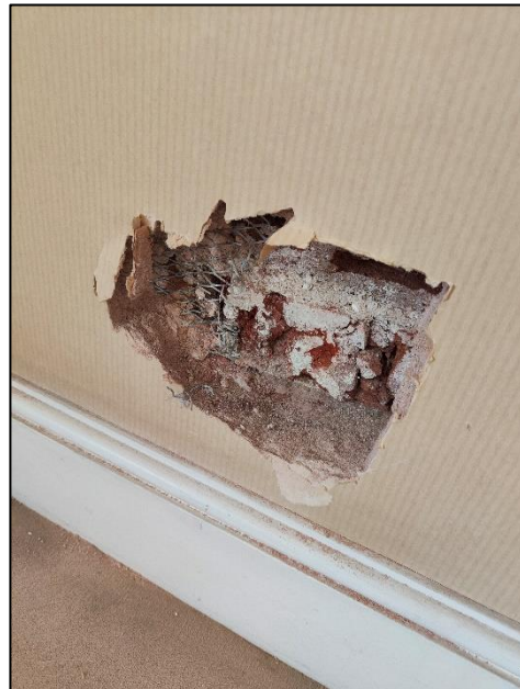
THIRD FLOOR TW2 Render on brickwork partition
