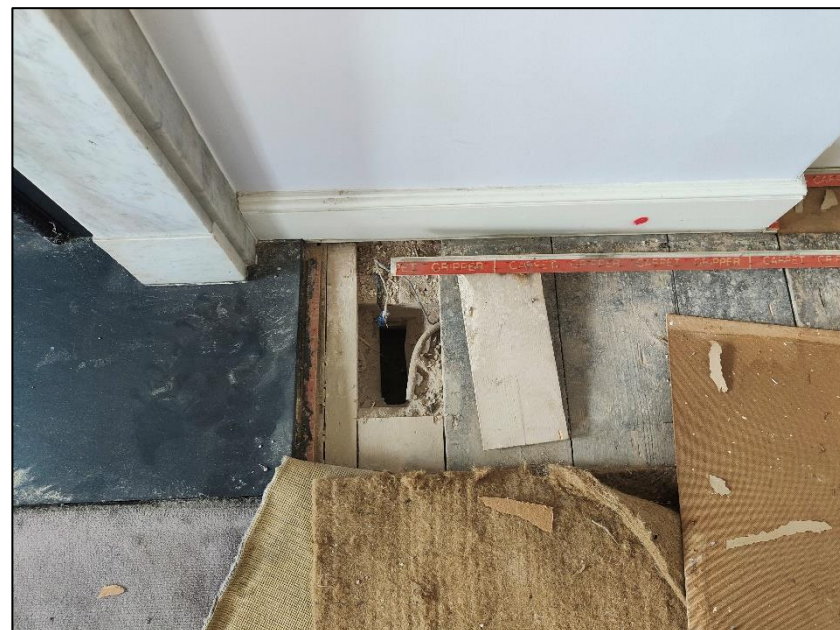
THIRD FLOOR T2 Timber boarding on timber joists
