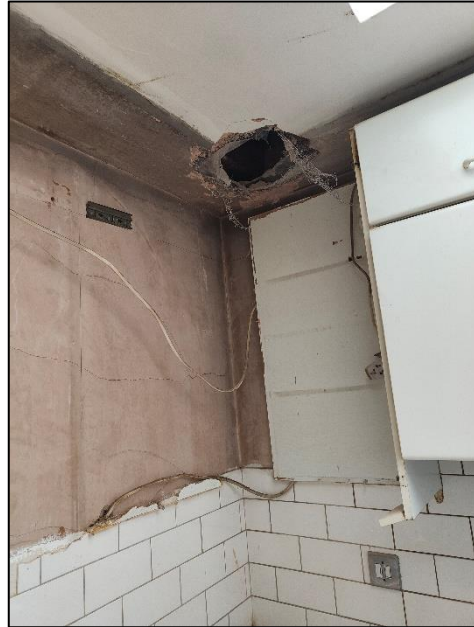
GROUND FLOOR GC1 Plasterboard ceiling on timber ceiling joists
