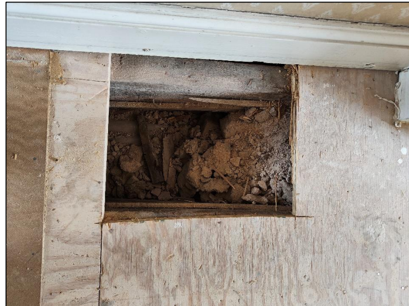
SECOND FLOOR S2 Timber boarding on timber joists
