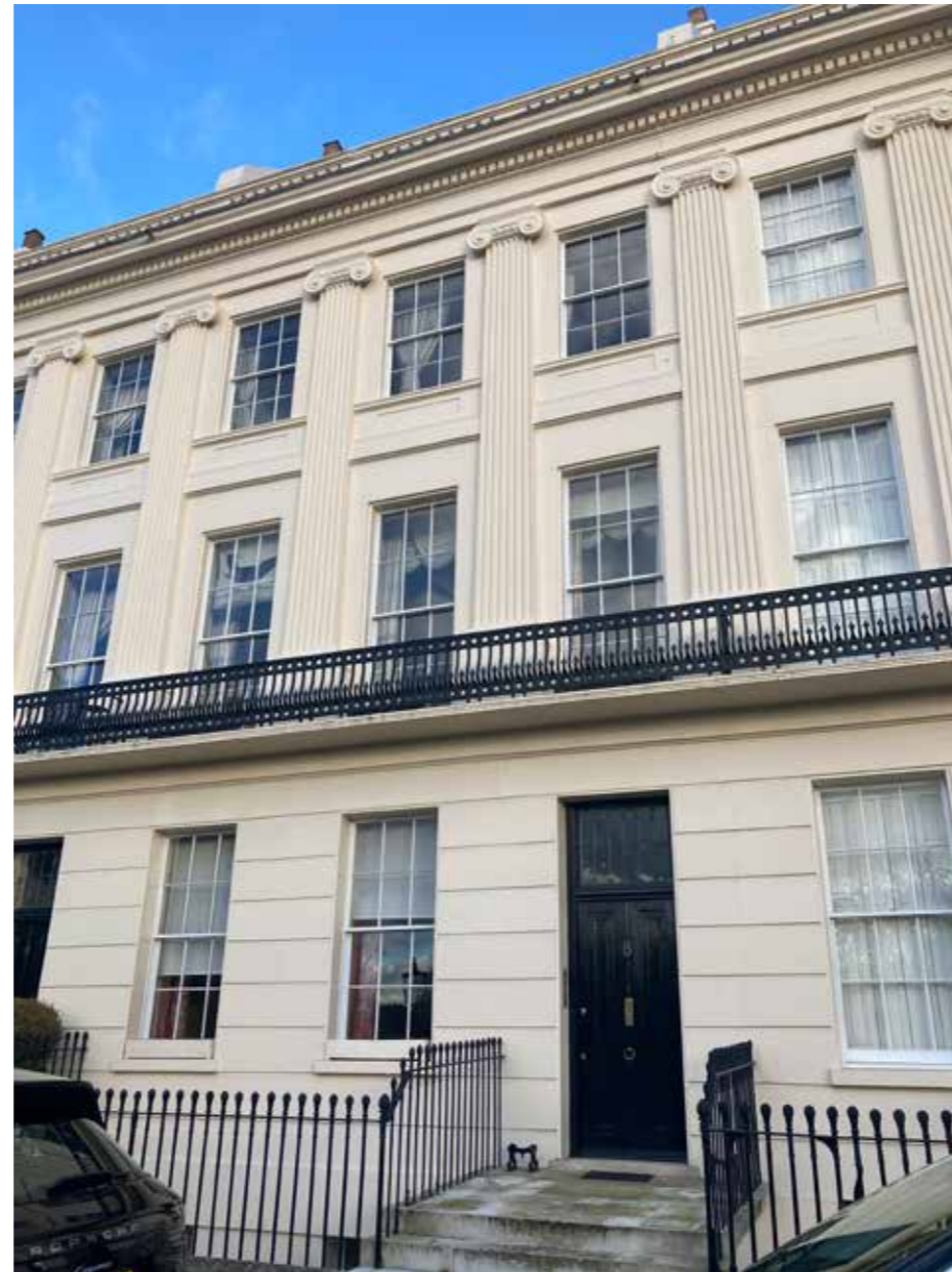
Figure 4.1 Principal elevation of 8 Gloucester Gate.
