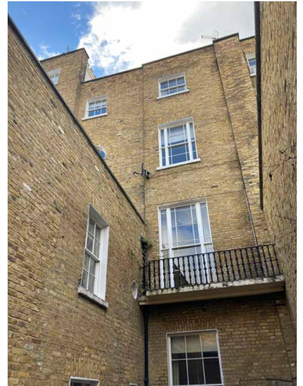
Figure 4.2 Rear elevation of 8 Gloucester Gate.
