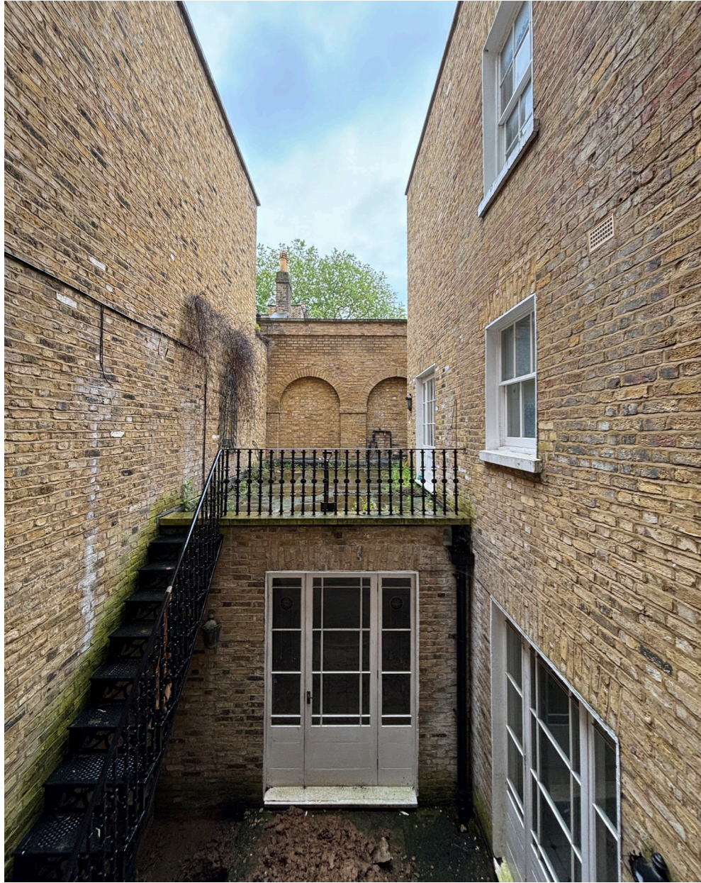
Experience of the courtyard looking from the main house principal floor
