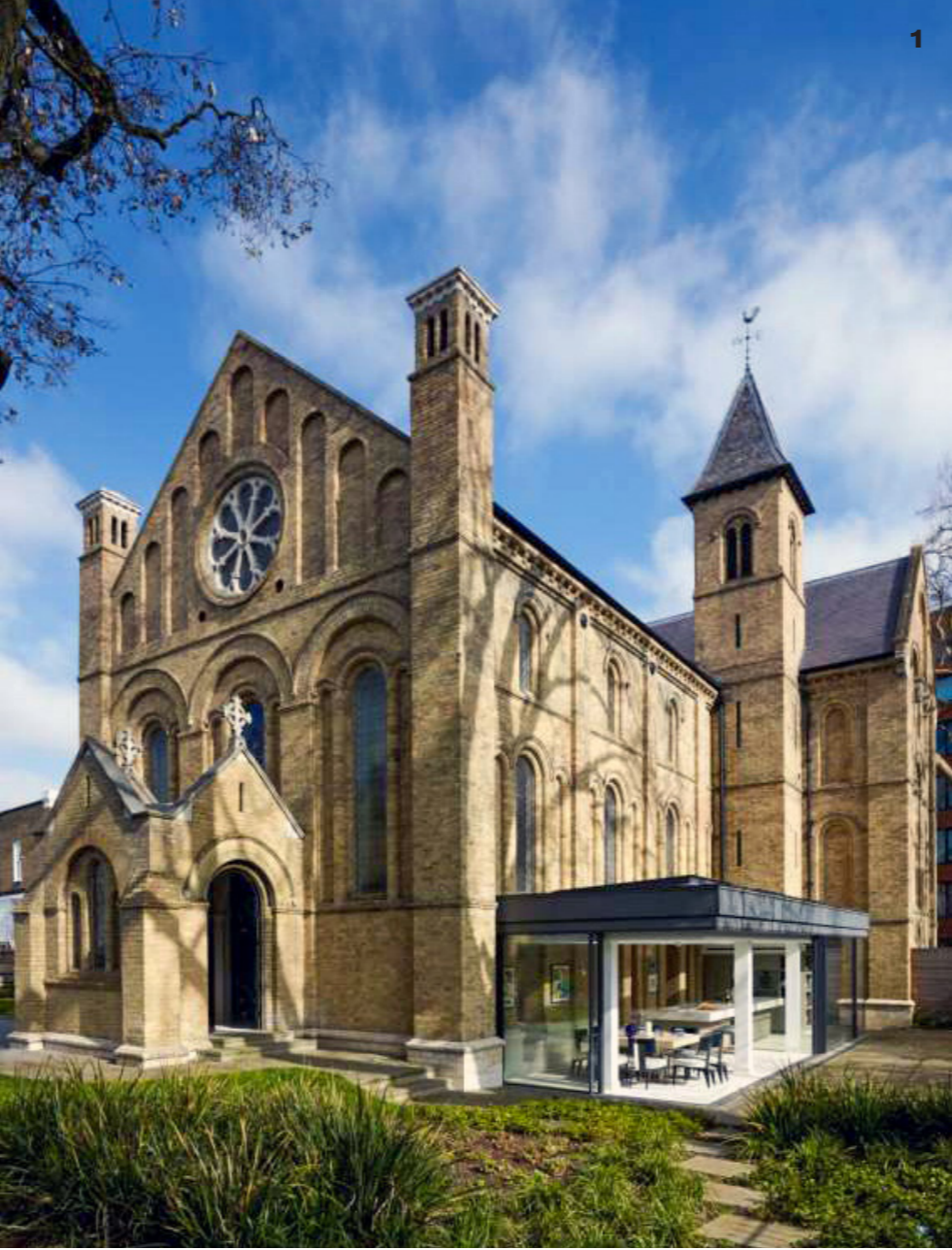
1 The King's Chapel, Chelsea: Adaptive re-use of a listed derelict chapel with a sensitive light touch approach to utilising its existing fabric .
