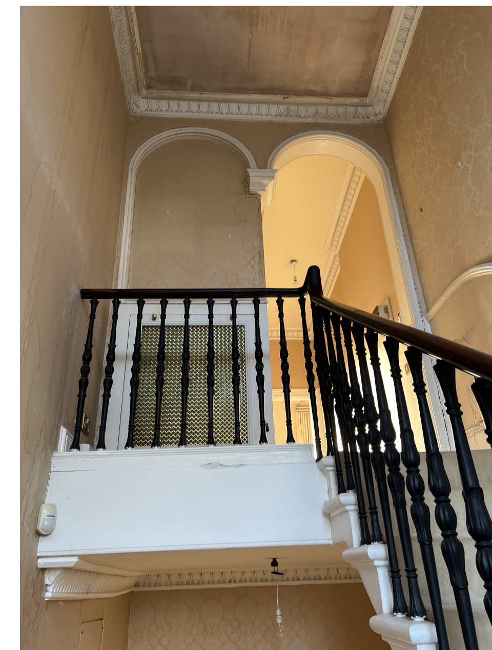
Existing arch condition
