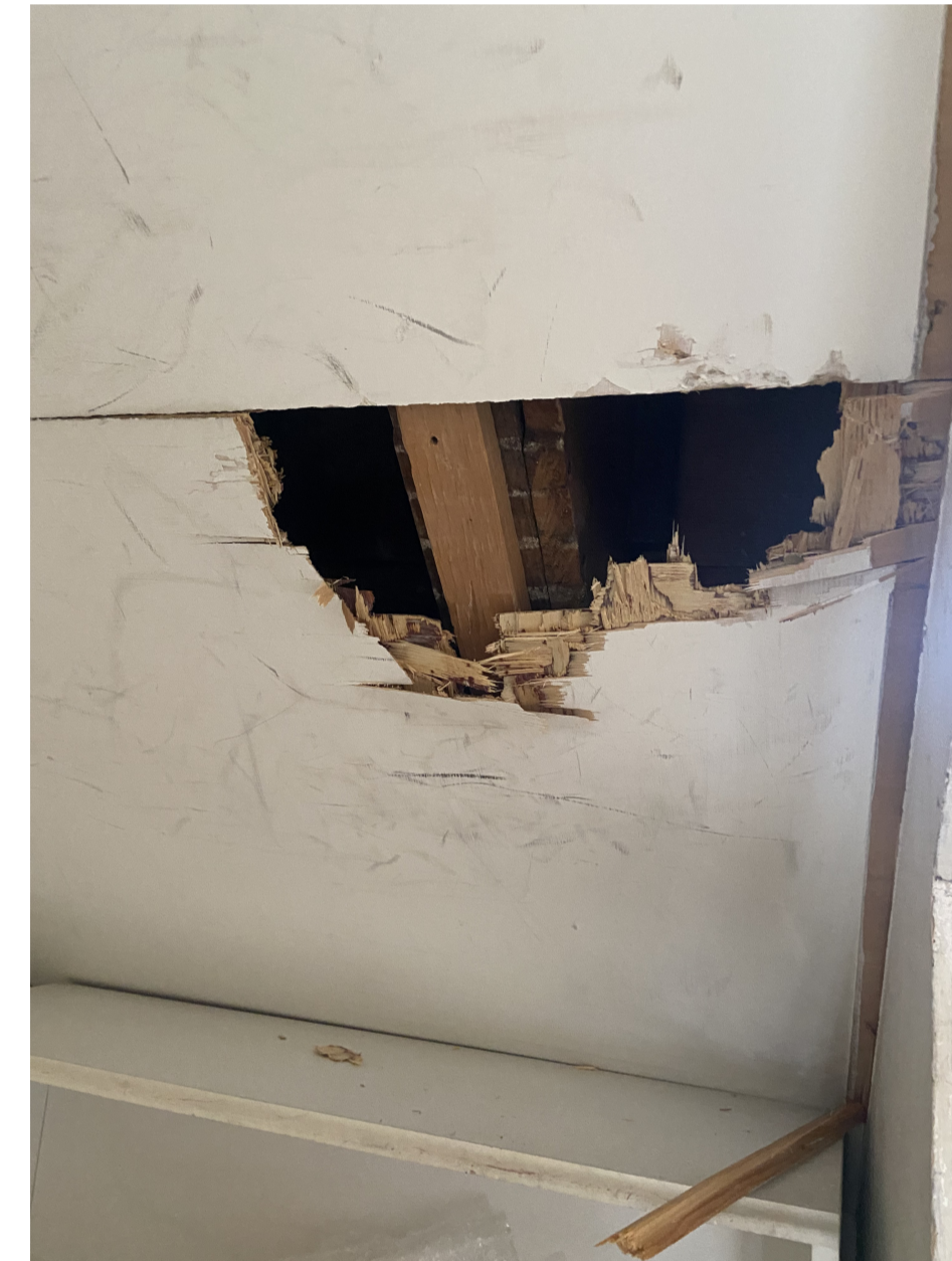
Existing stair condition
