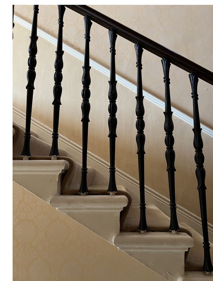
Existing stair condition
