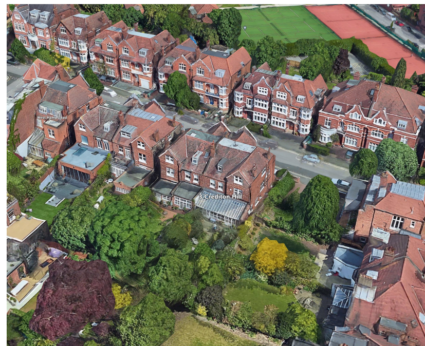
REAR AERIAL VIEW
