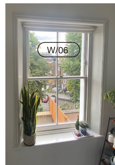
Existing Windows Interior
