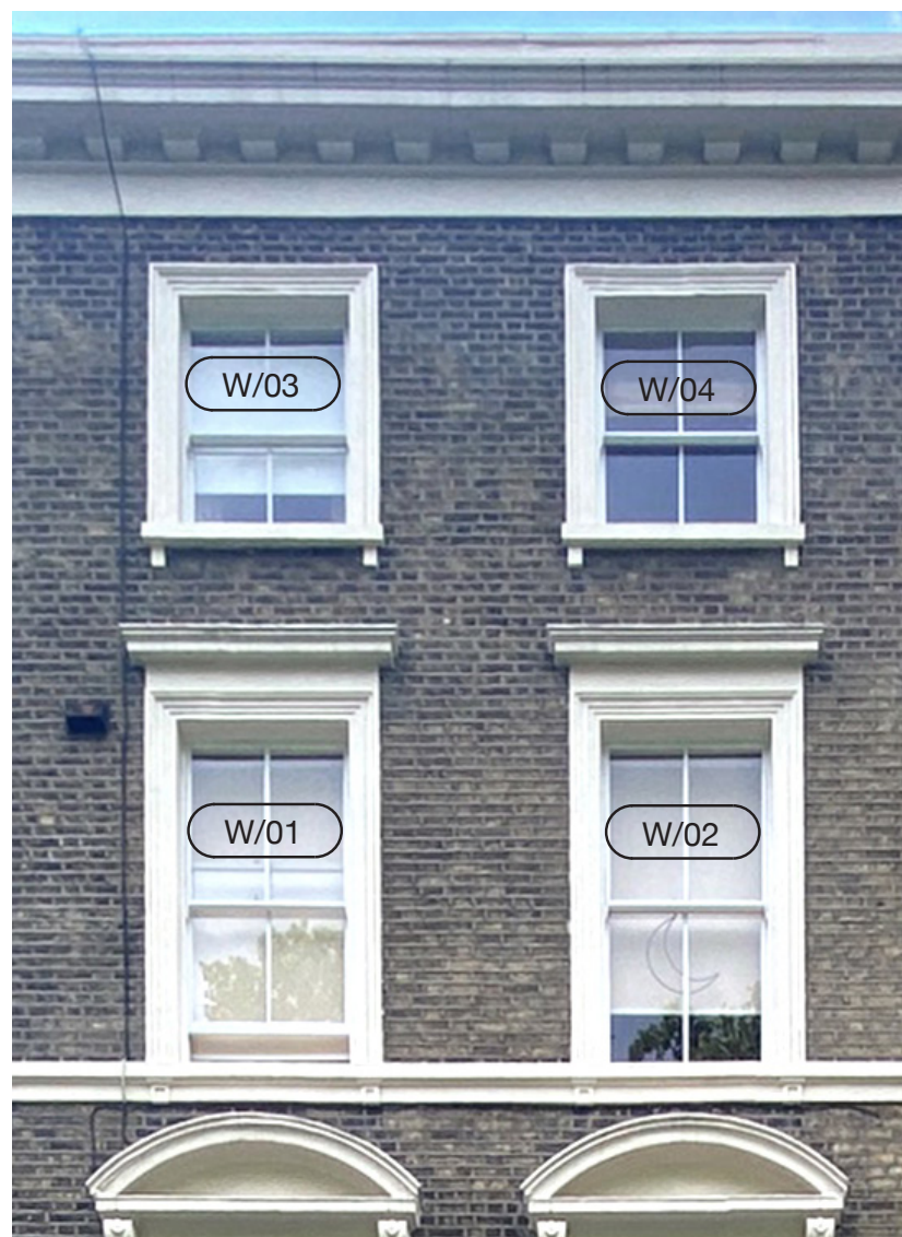
Existing Windows Front Elevation
