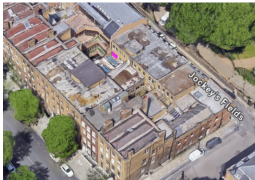
Figure 3: Ariel view showing position of the window to be blocked on the rear façade of the 1960s Jockey field building (window shown in pink)
