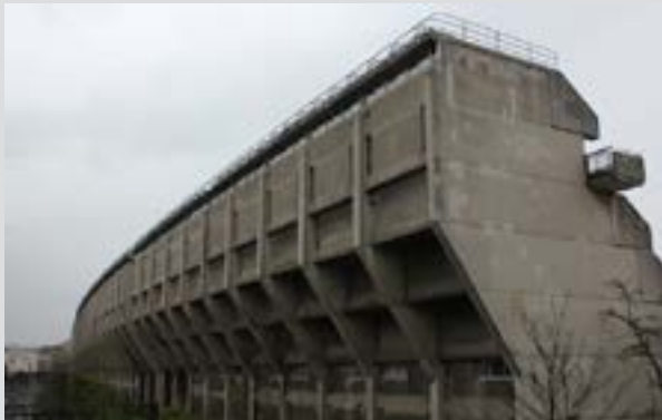
Alexandra Road Estate, Neave Brown (1972-78)
