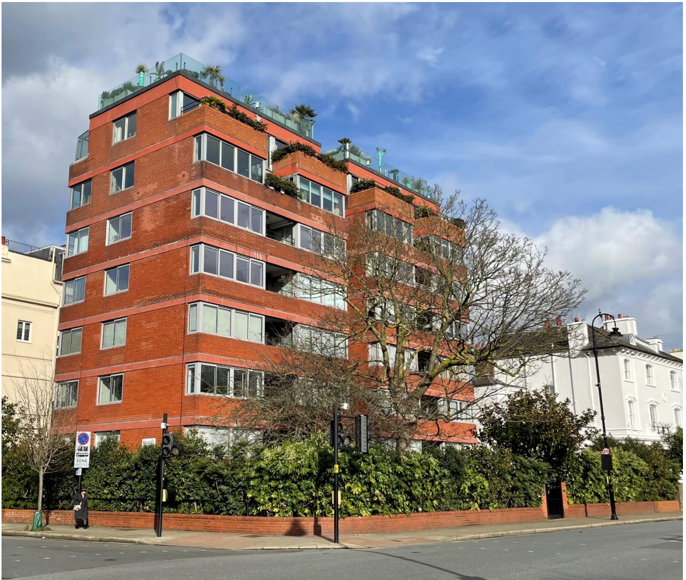
Figure (a): View of front and side elevation of appeal site from Prince Albert Road.
