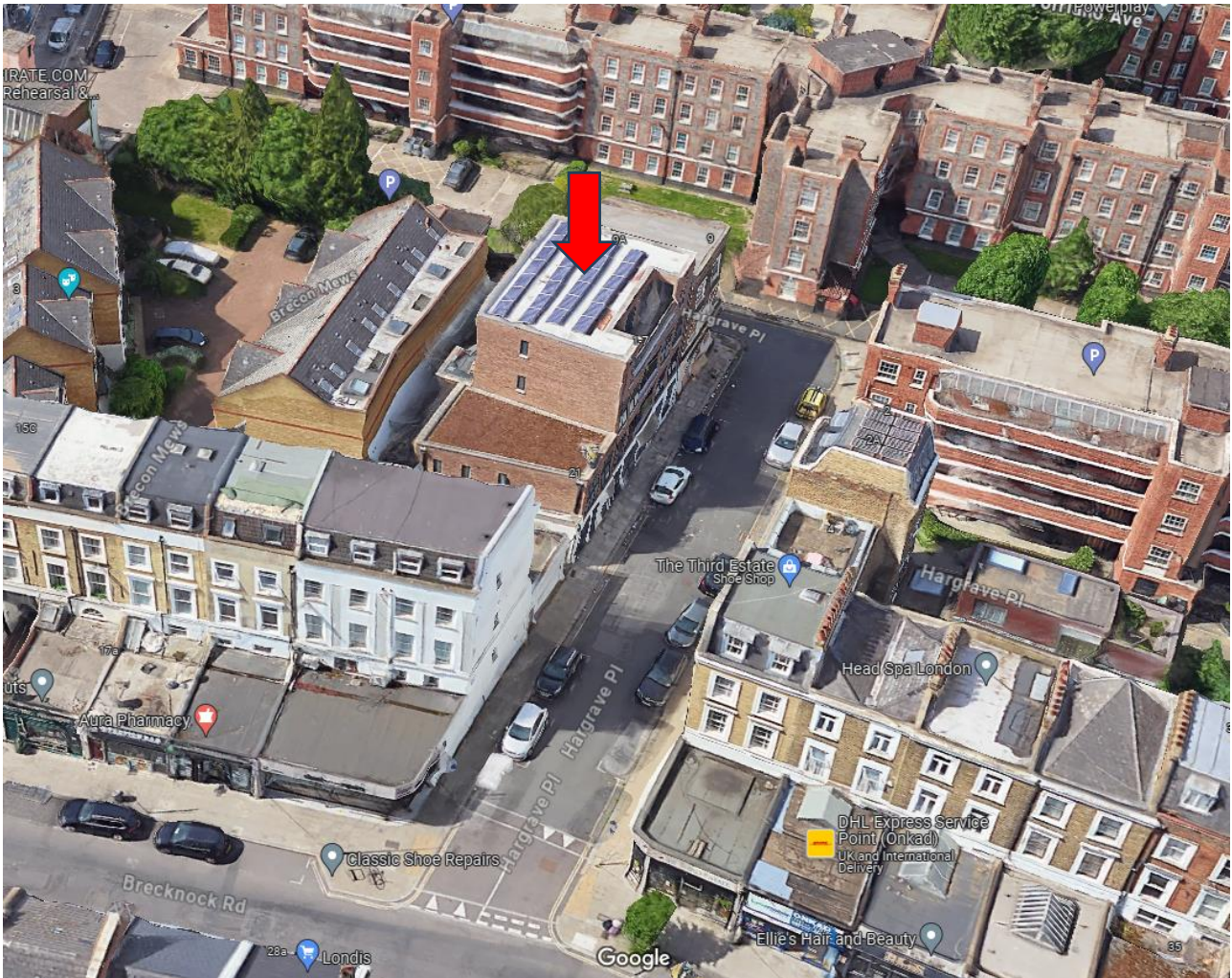
Figure (a): Aerial view of the appeal site in context (source: Google 3D)
