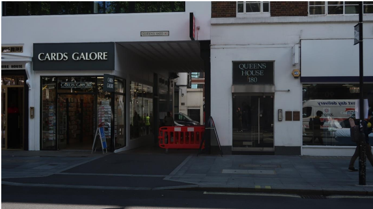
Image 1: view of the existing entrance door to the Queens House at No.180 Tottenham Court Road
