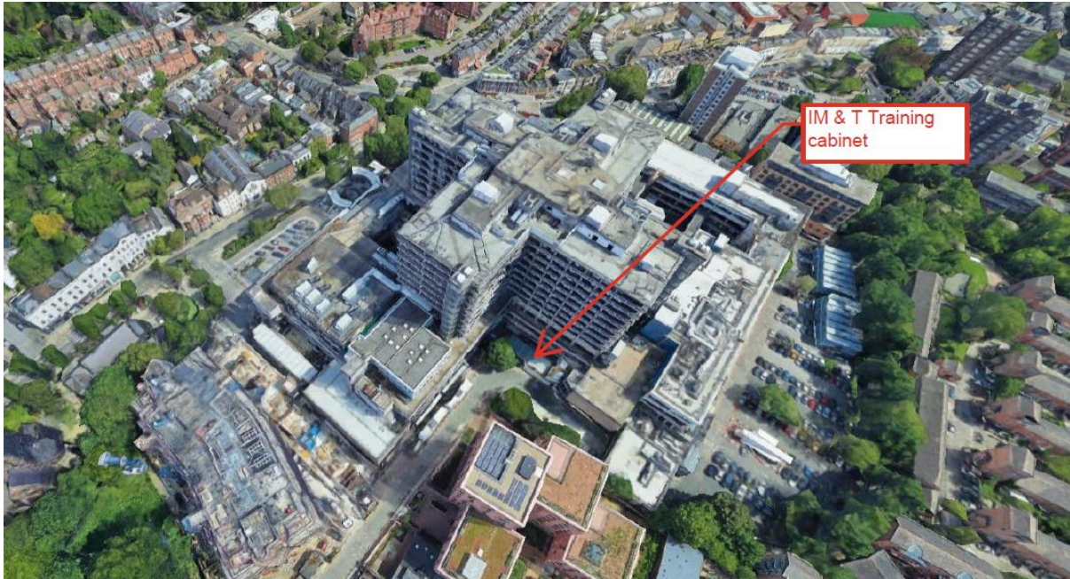
Image 5. Existing IM & T training cabinet. Aerial view
