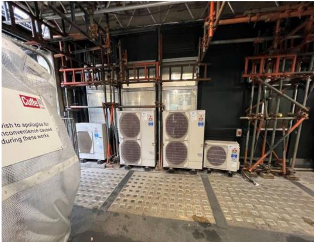
Image 9. 4no. units to be relocated.
