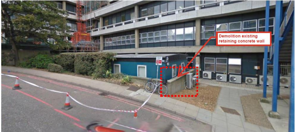
Image 7. Existing retaining wall to be demolished.
