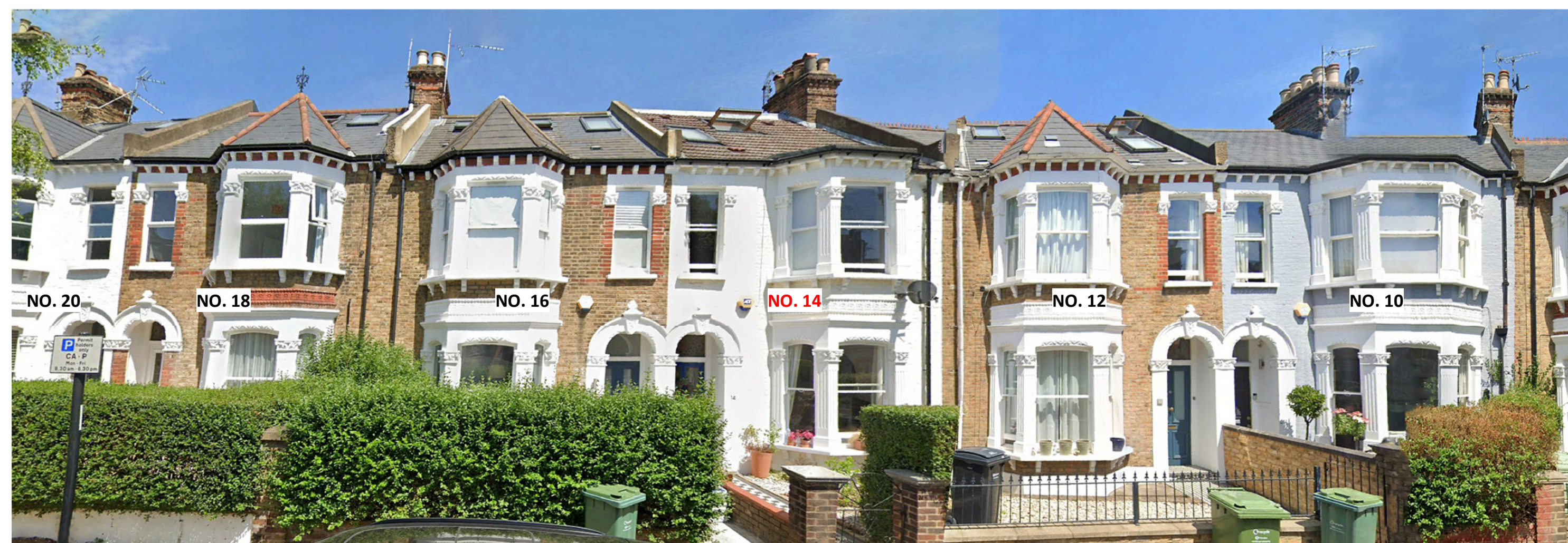
IMAGES OF EXISTING - SOUTH ELEVATION LOOKING AT 14 SOLENT RD WITH 10 & 12 SOLENT RD TO THE RIGHT AND 16, 18 & 20 SOLENT RD TO THE LEFT.
