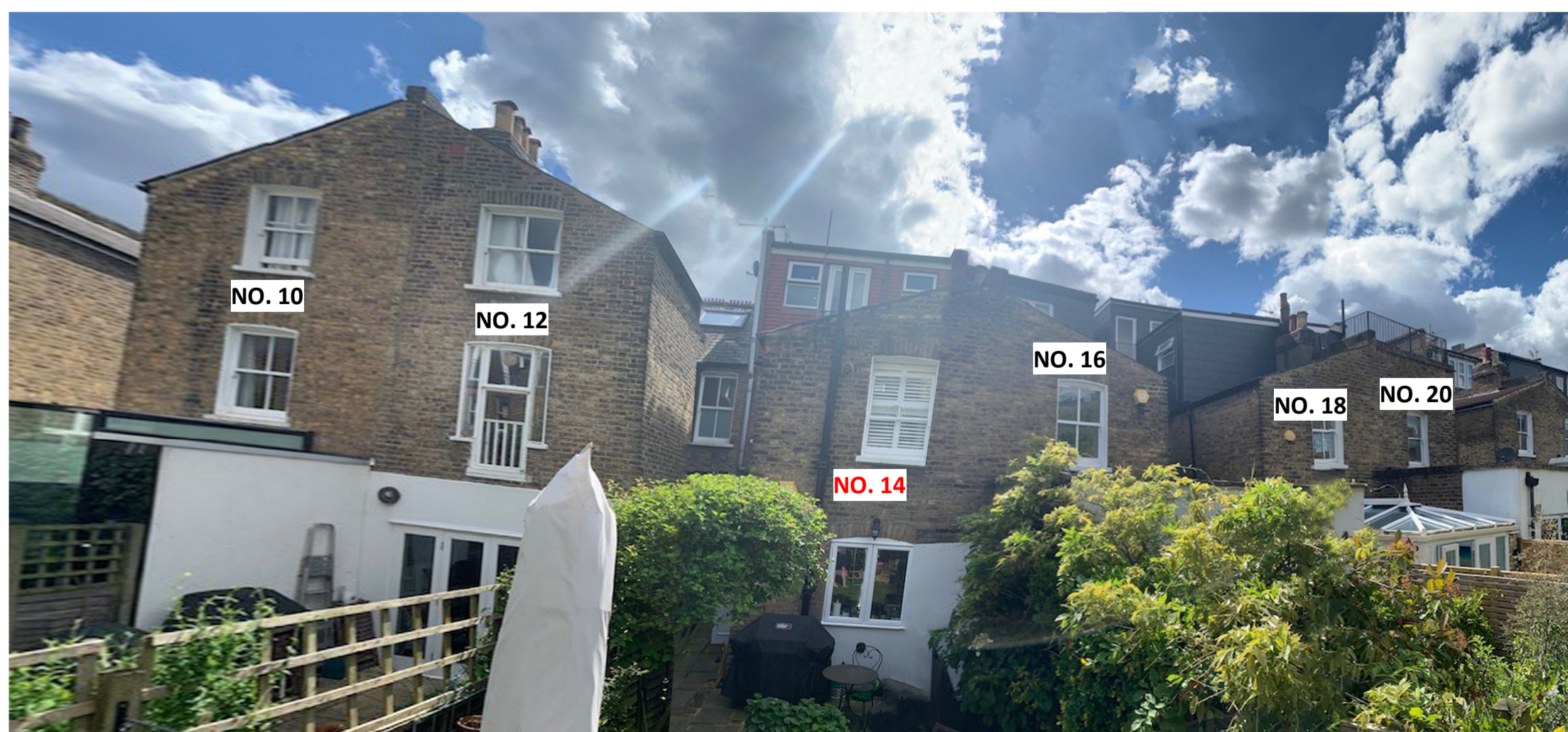
IMAGES OF EXISTING - NORTH ELEVATION LOOKING AT 14 SOLENT RD WITH 10 & 12 SOLENT RD TO THE LEFT AND 16, 18 & 20 SOLENT RD TO THE RIGHT.
