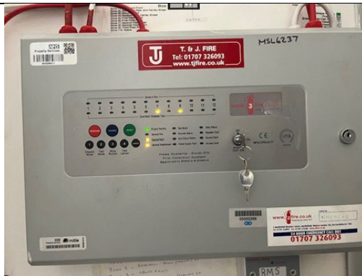
Existing Fire alarm panel
