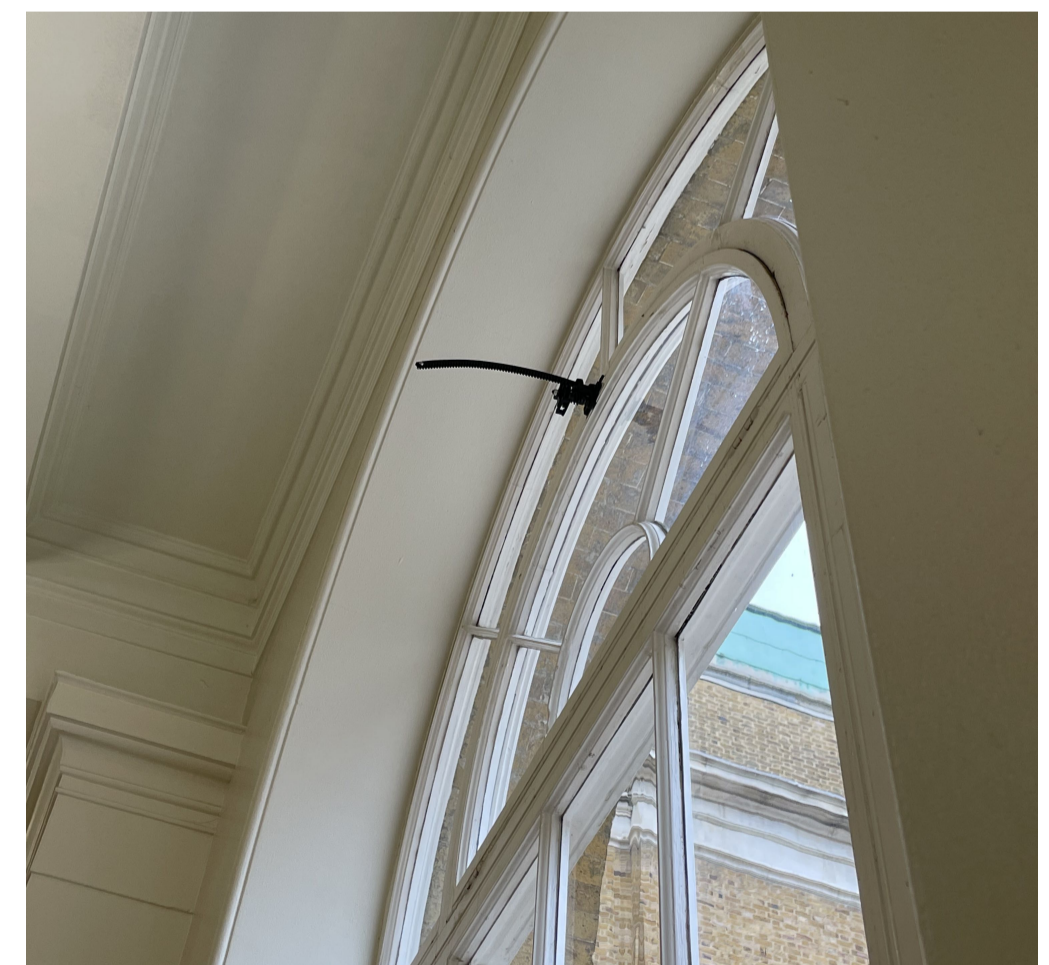
Existing quadrant fanlight arm stay
