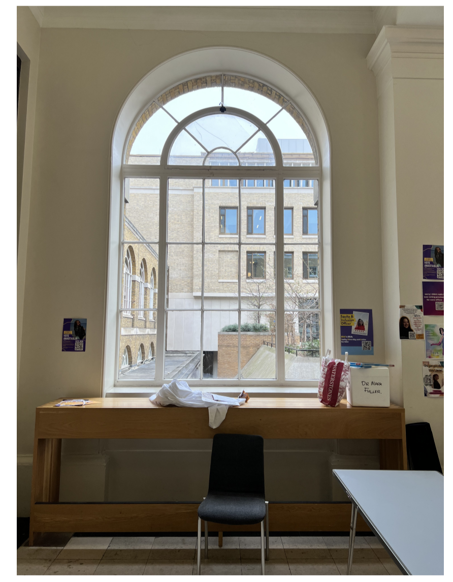
Existing cloisters window (with openable panels)
