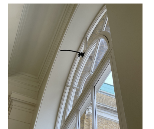
Existing quadrant fanlight arm stay
