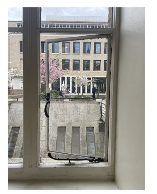
Existing openable panel
