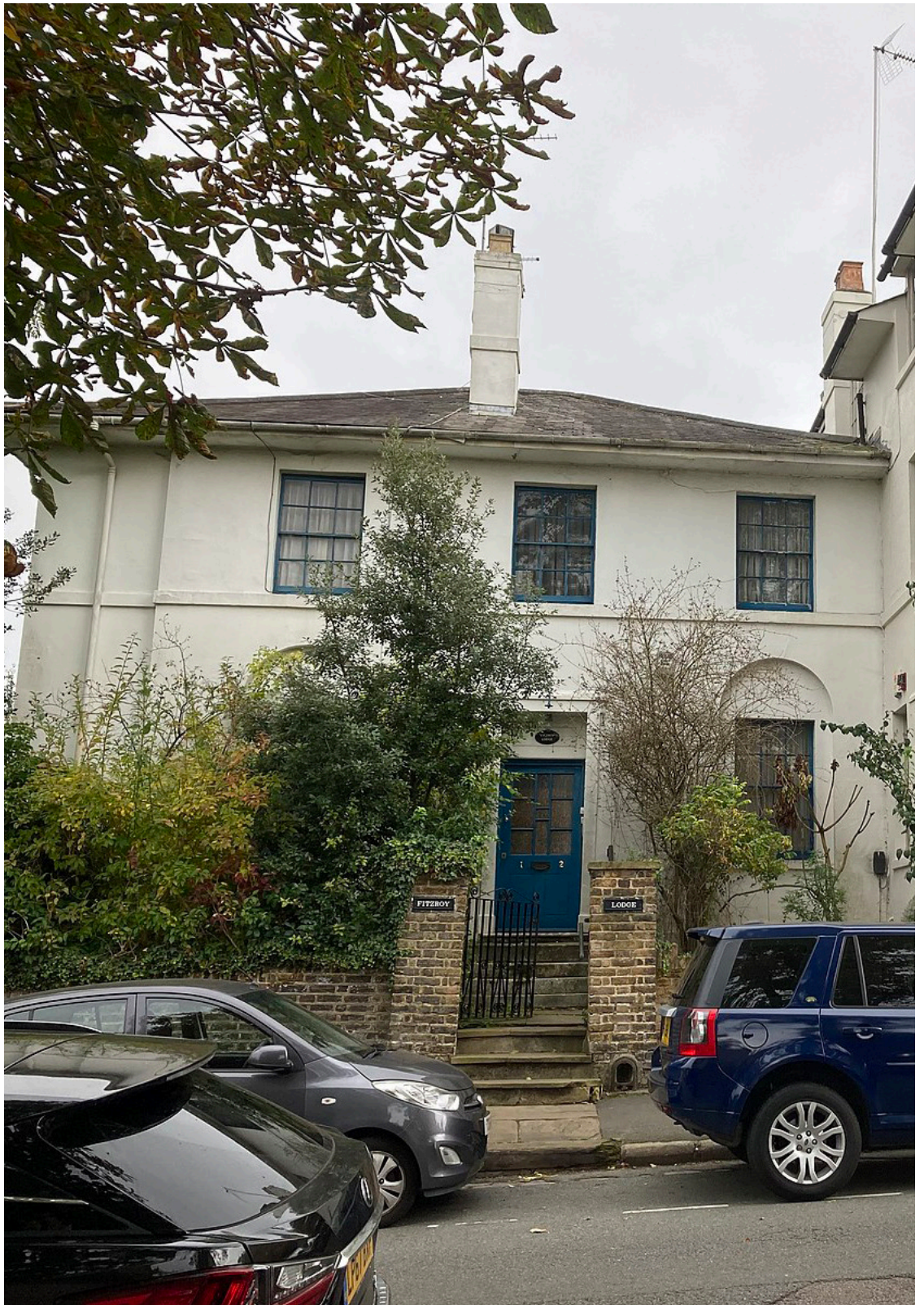
Street view of Flats 1 & 2 Fitzroy Lodge, N6 6LH
