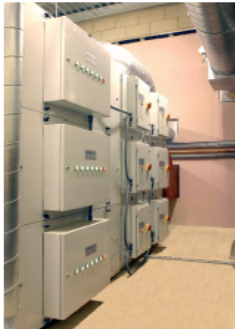
Six ESP and Three UV-C modules installed as an integrated system.
