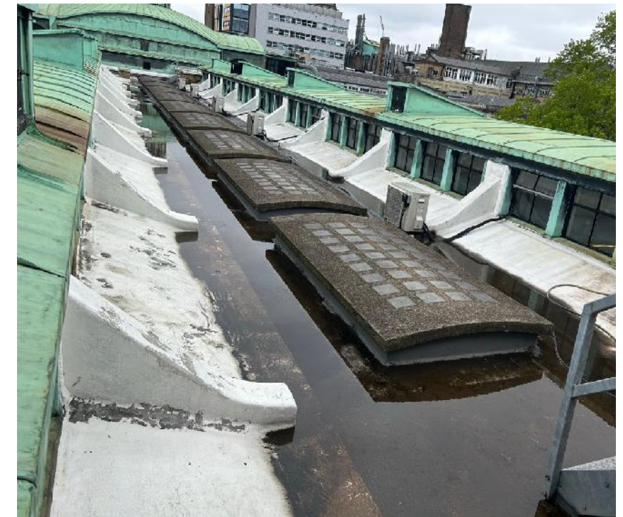
Photograph of South Cloister roof
