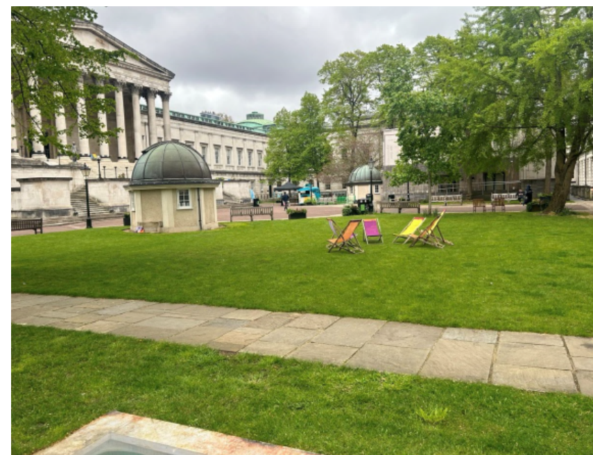
Photo showing structures within Quad
