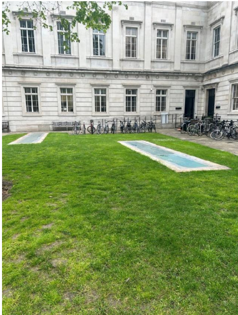
Slade basement roof lights
