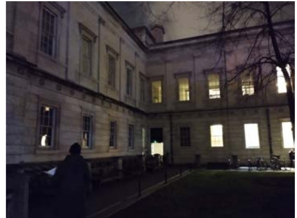
Areas with no spill light from the windows were visibly darker than areas with internal illumination switched on. The resultant high contrast is hazardous.
