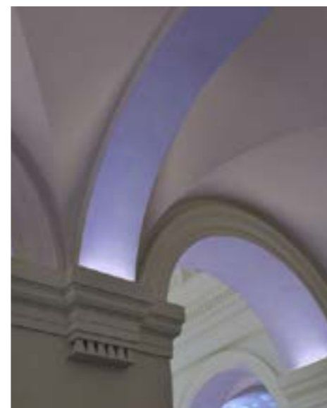
Opportunity for RGB lighting within cornice detail
