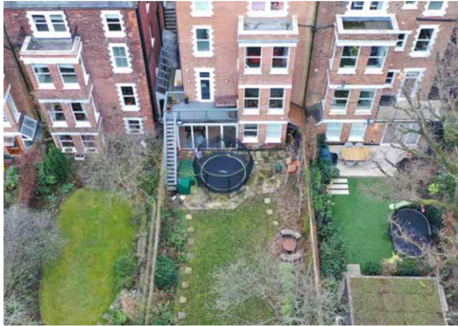
↑ No. 21 Tanza Road - large rear extension
