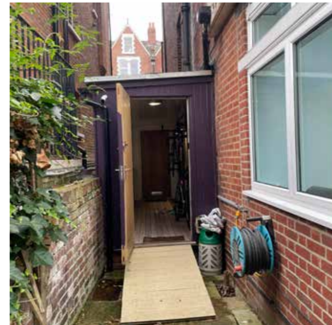
↑ Existing side extension seen from rear
