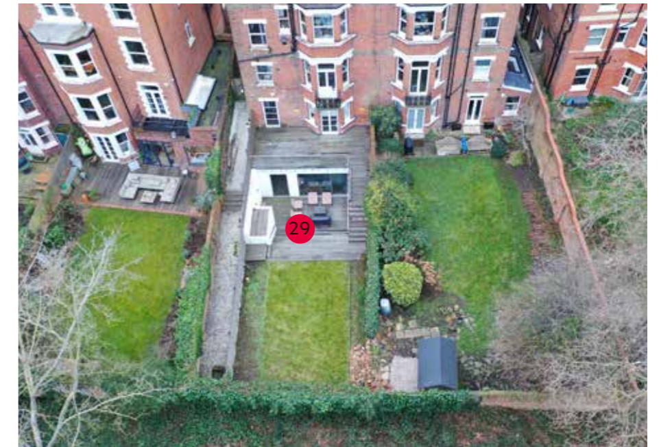
↑ No. 29 Tanza Road - extensive lower ground floor excavation and full width terrace extension at ground floor
