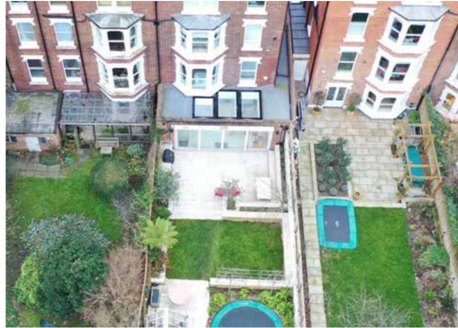
↑ No. 3 Tanza Road - full width rear extension
