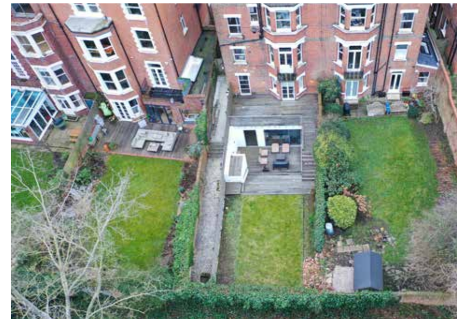
↑ Rear of No.29, showing full width rear extension
