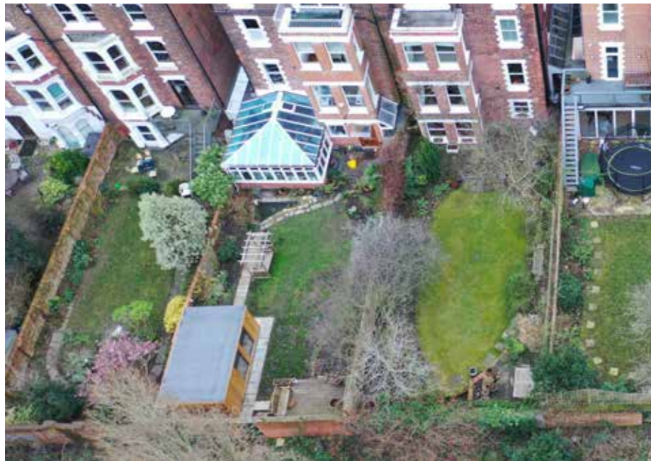
↑ No. 17 Tanza Road - large rear extension and alterations to existing bay fenestration
