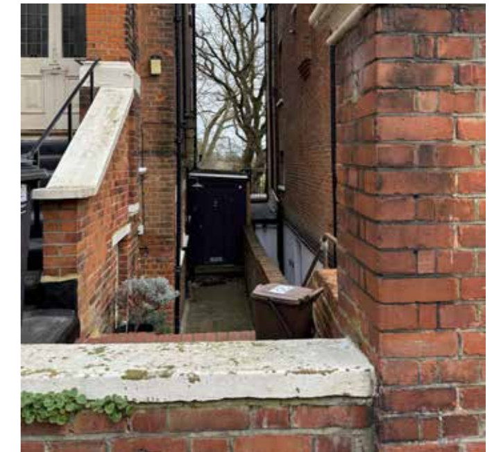
↑ Existing side extension seen from street
