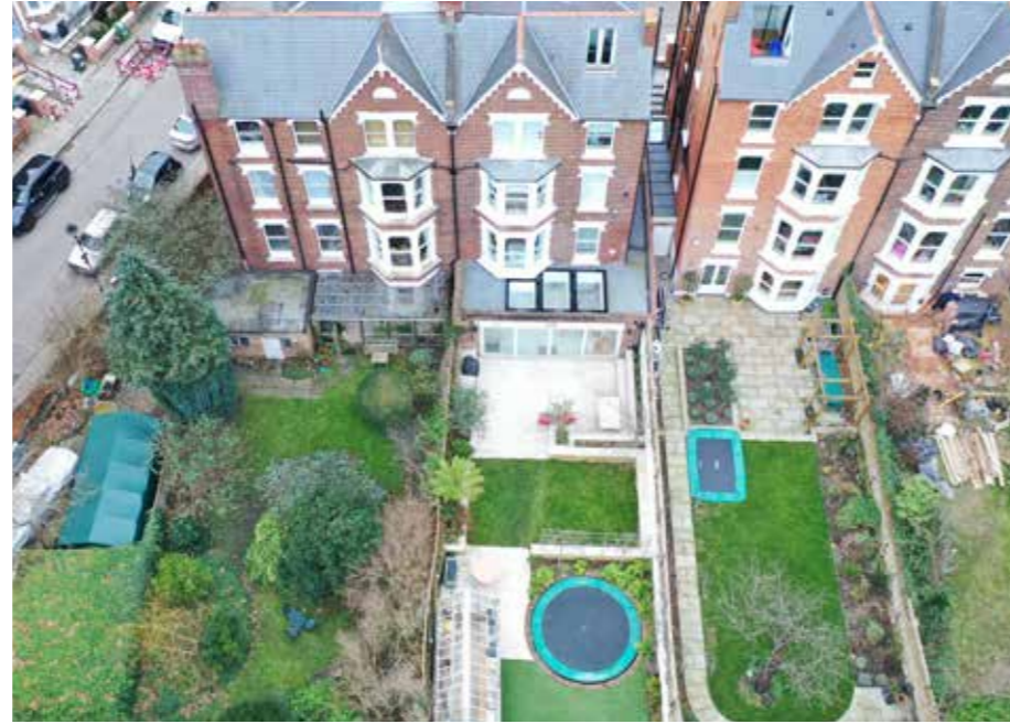
↑ Rear of No.3, showing full width rear extension
