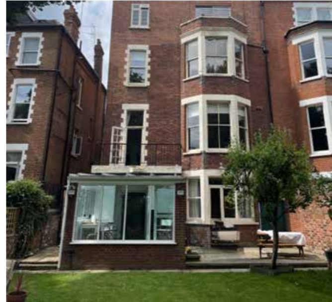
↑ Existing conservatory extension and rear of building
