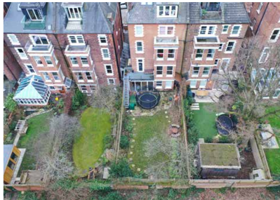
↑ Rear of No.21, showing rear extension.
