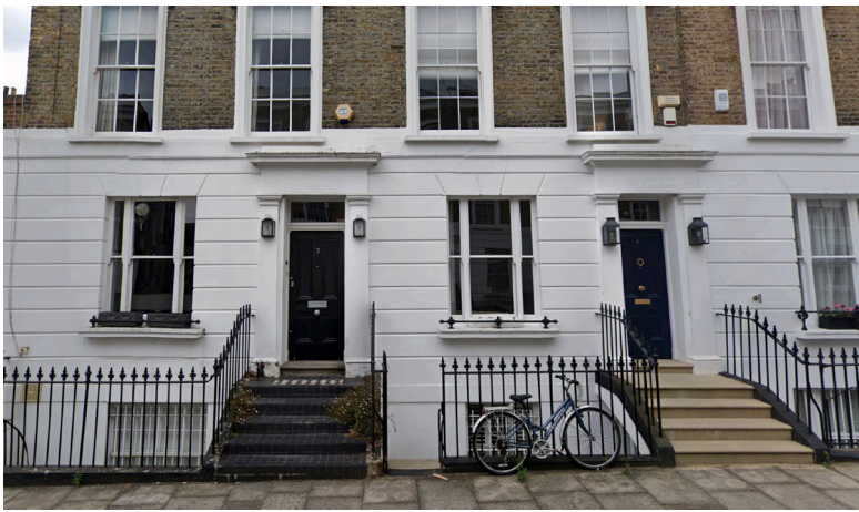
External wall light to the pilasters flanking the entrances to No. 6 & No.7 Rothwell Street
