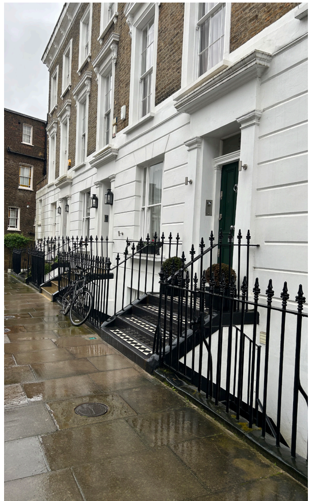
External wall light to the pilasters flanking the entrances to No.5 No.6 & No.7 Rothwell Street.
