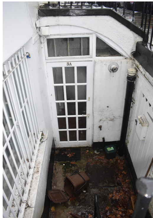
Front area showing modern infill to understairs area. Existing basement window has been enlarged.
